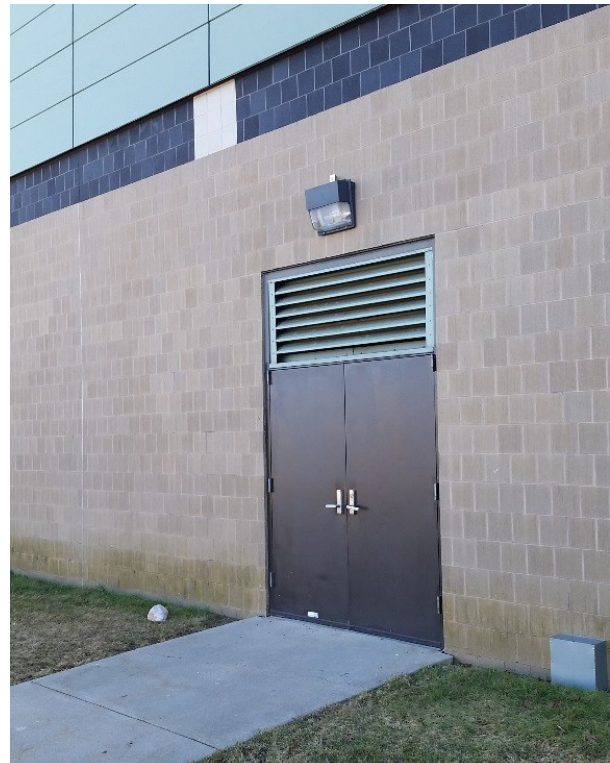
Electrical Photograph #11 Exterior light with photocell at 1990 Gym Addition
