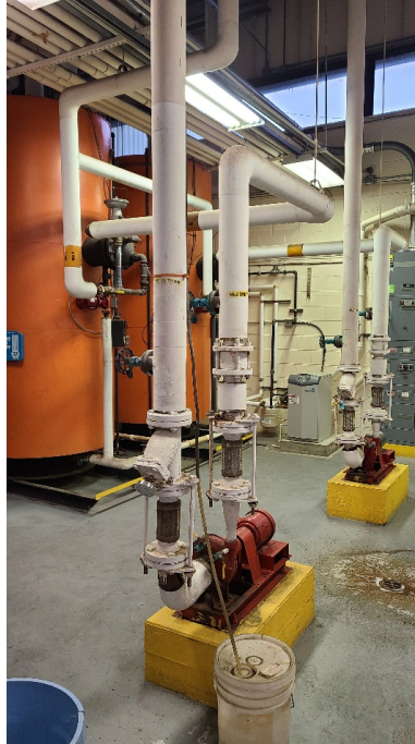
Figure 4: Domestic Hot Water System
