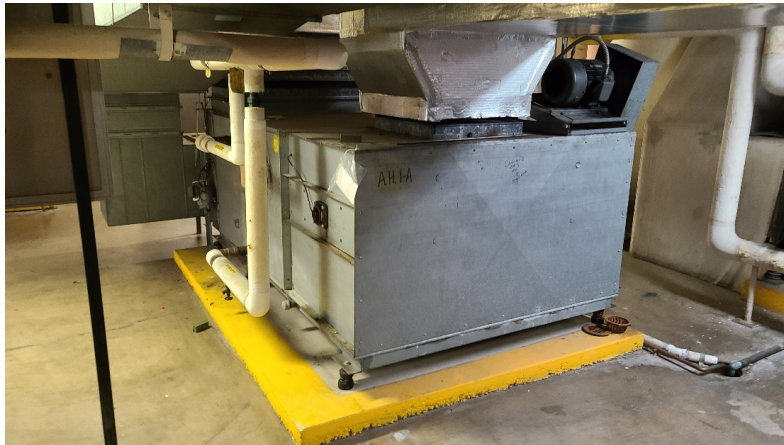
Figure 7: Typical Air Handling Unit
