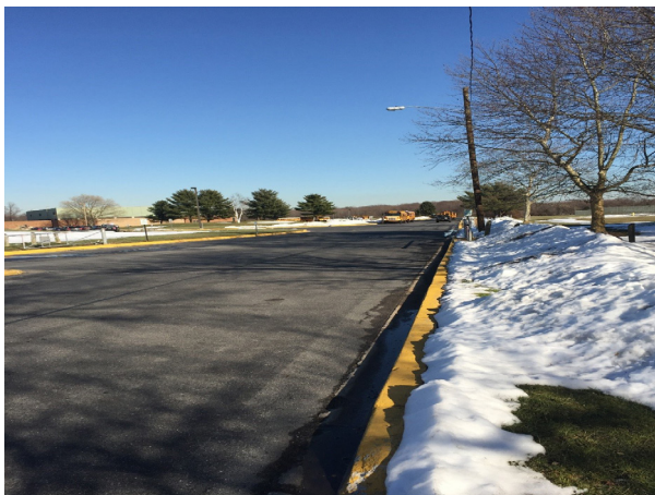
Figure 2.4 Main Access Road on site looking east.
