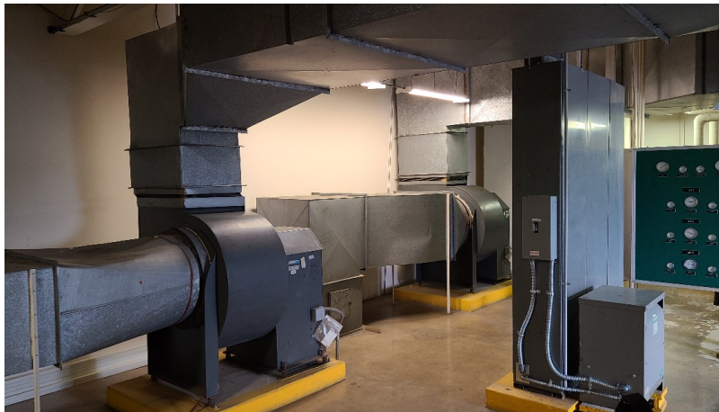
Figure 6: Typical Return Fan
