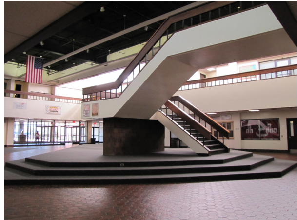
Figure 1.3 Non-Code Compliant Issues Throughout
