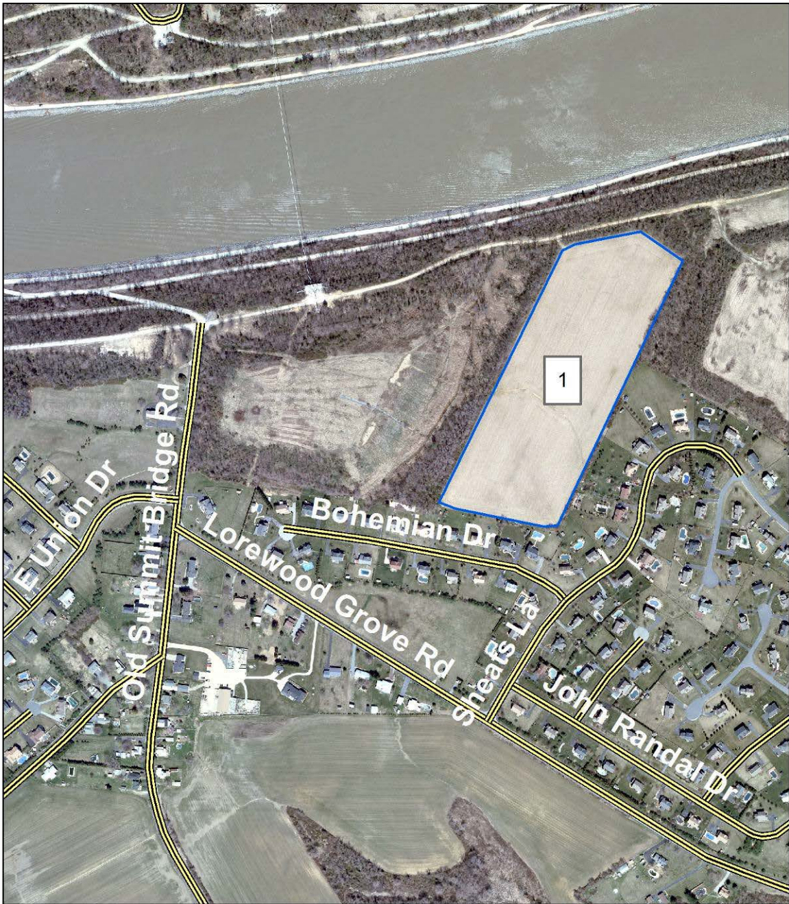
Exhibit 2. Aerial view of C&D Canal Conservation Area – Summit Tract near Middletown, Delaware.
