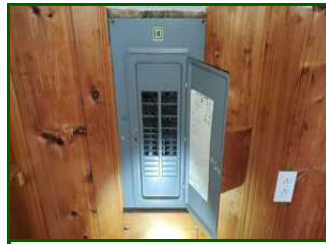
Location: 3RD FLOOR
