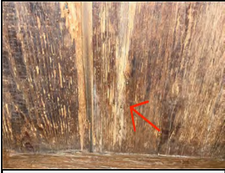
Termite damage
