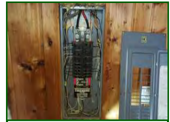
Location: 3RD FLOOR
