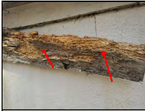
Termite damage
