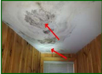
Location: 3RD FLOOR
