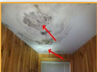
Location: 3RD FLOOR
