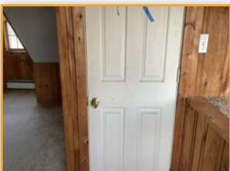
Location: 3RD FLOOR
