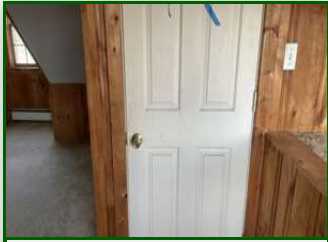
Location: 3RD FLOOR
