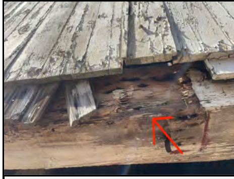
Termite damage
