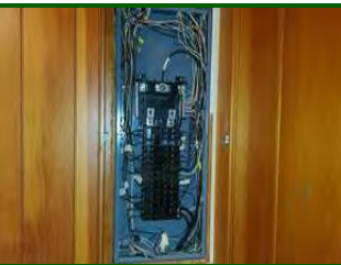
Location: STUDIO GARAGE
