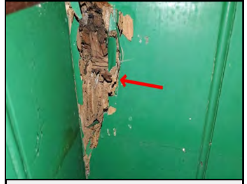
Termite Damage
