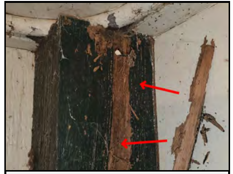
Termite Damage
