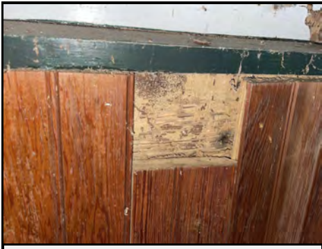
Termite damage
