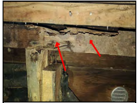
Termite Damage
