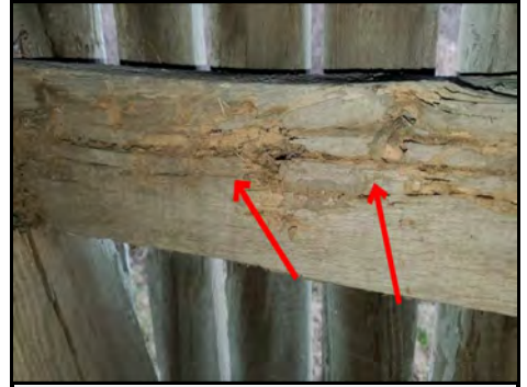
Termite Damage
