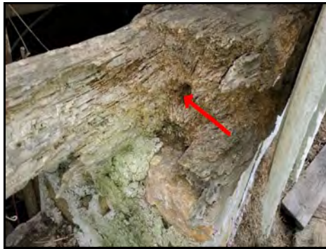
Termite Damage
