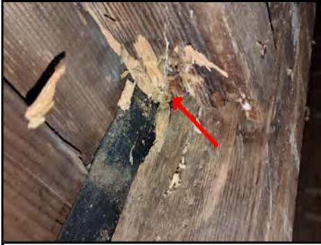
Termite Damage
