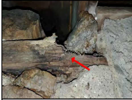
Termite Damage
