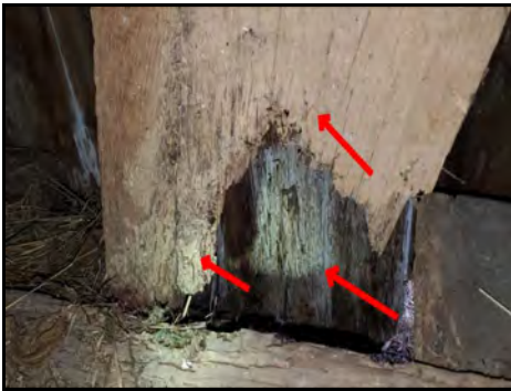
Termite Damage
