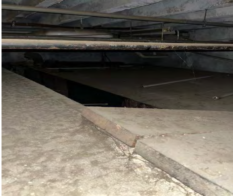
Top of tank looking southwest.
