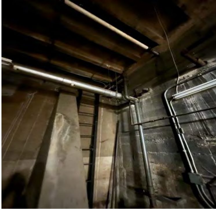
Southeast vault detail with boiler room wall to right
