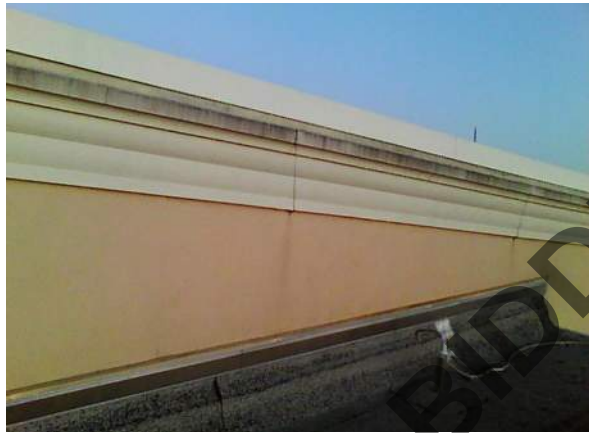
Façade Photos Daytime
