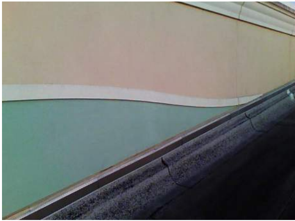
Façade Photos Daytime
