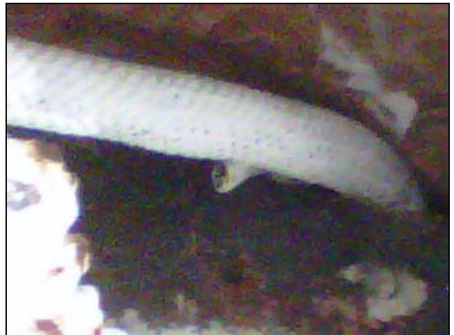
Remnant coated electrical wiring.
