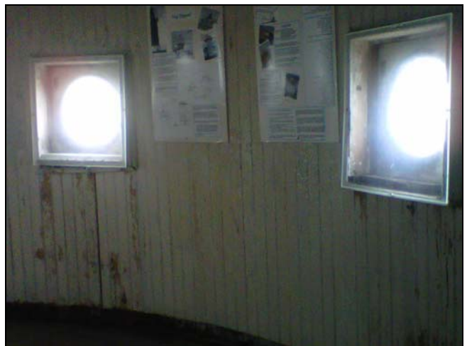
Upper Level wall and windows.
