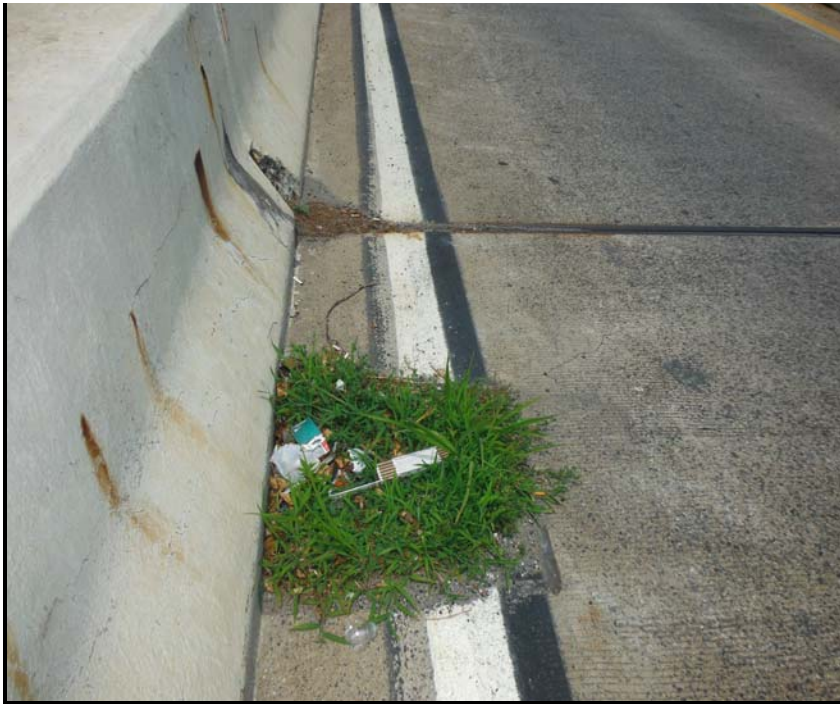
7. Span 5B, scupper is completely clogged with vegetation.
