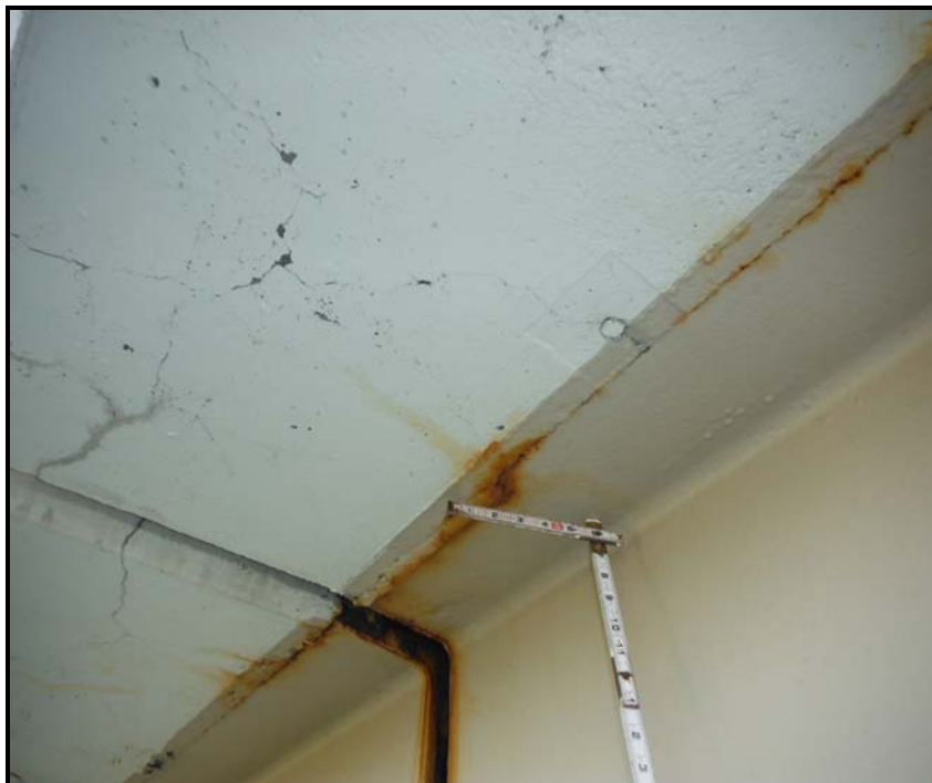
10. Span 6B, Beam 1, TF at N. End - Exp. and rusted steel.
