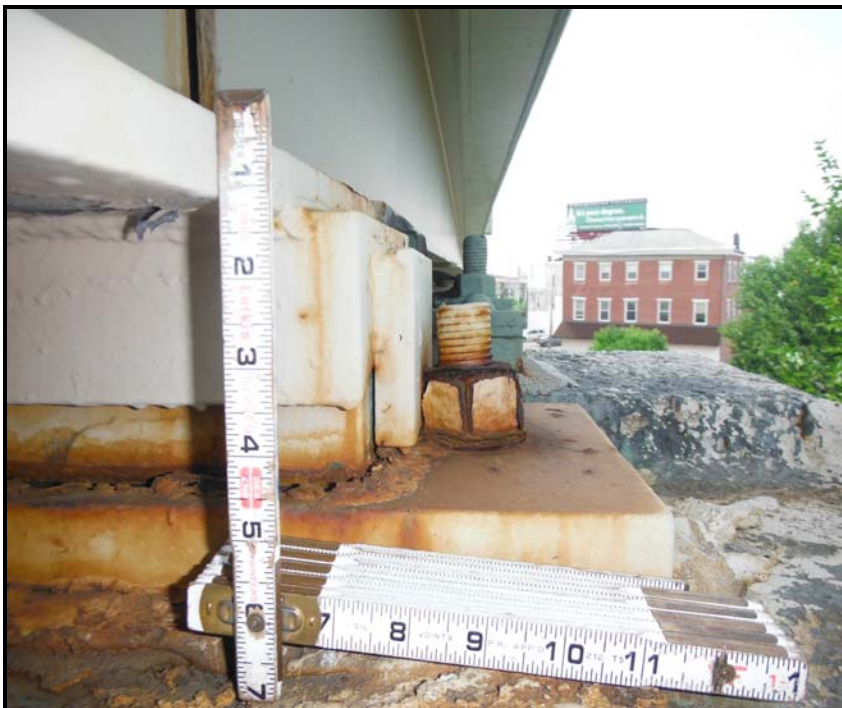
12. Pier 5B, Bearing 1 - W. Anchor Bolt is rubbing against bearing.
