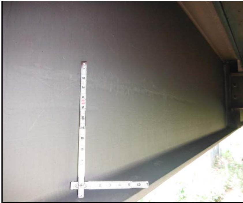
9. Span 1B, Beam 1 @ N. End - 6' L x 2" H x 1/16" D SL in web.
