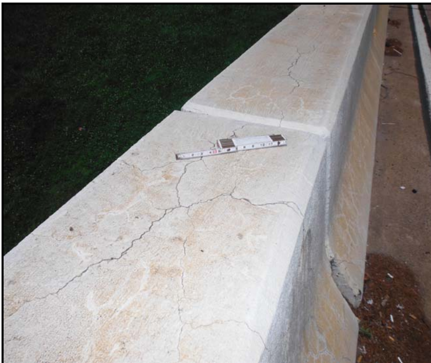
8. Span 2, West Parapet - HL to 1/16" wide map cracking.
