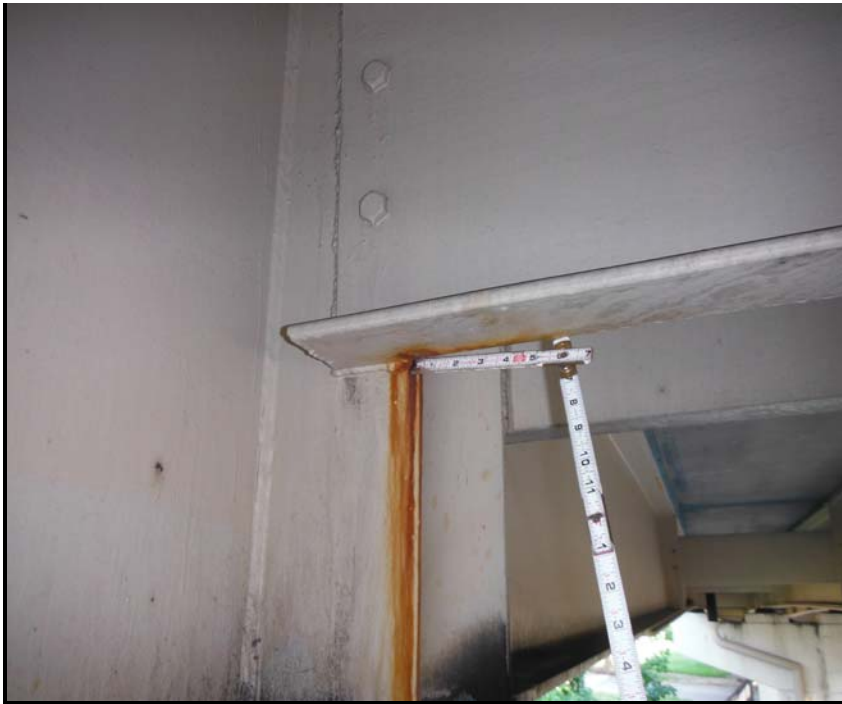
11. Span 6B, diaphragm over Pier 6B - Exposed and rusted steel.
