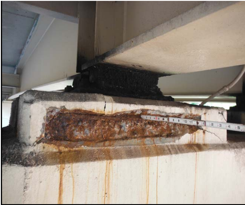
13. Pier 4B, Ped. 2, N. Face - 3' L x 6" H x 2" D spall w/ exp. rusted steel.
