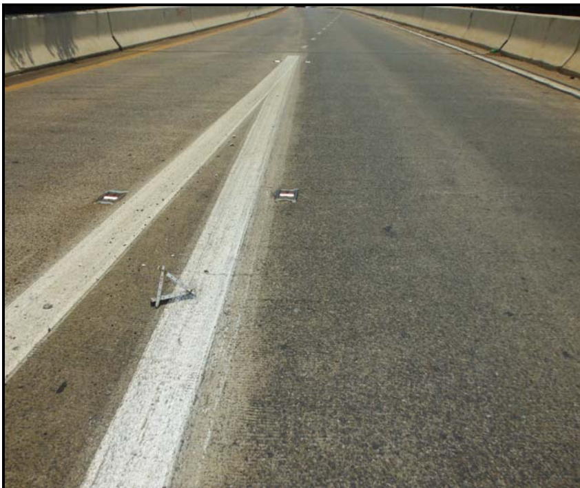
6. Typical condition of deck with moderate wear (Span 2B shown).
