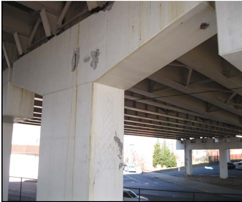
17. Large open and incipient spalls in the cap and stem of Pier 6, looking Northwest
