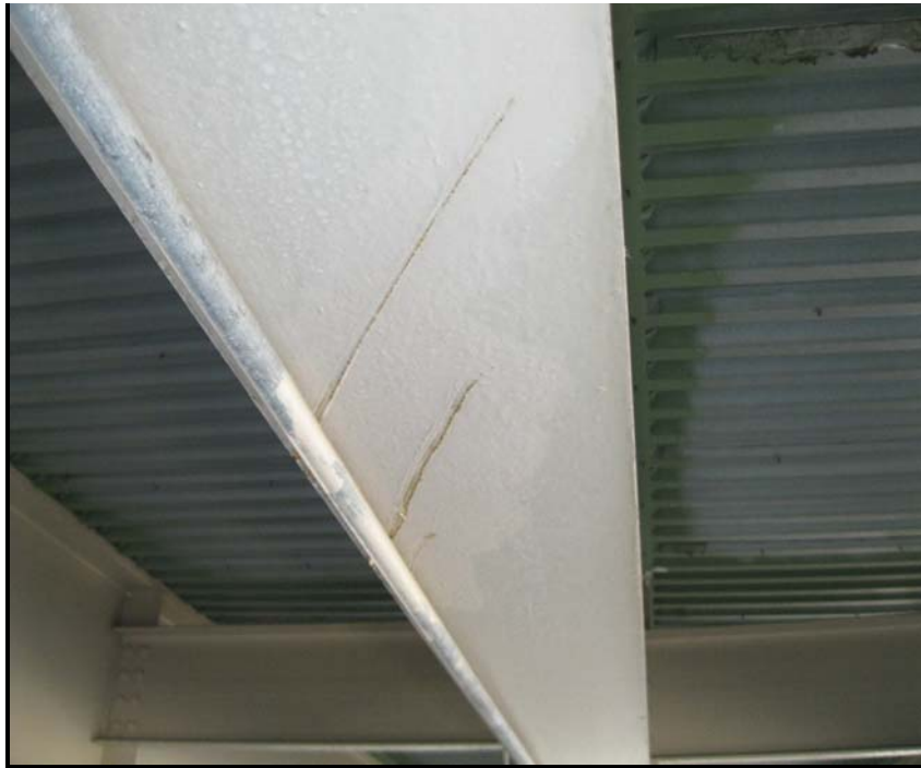
15. Scrapes and gouges with rust in the underside of Beam 3 in Span 9
