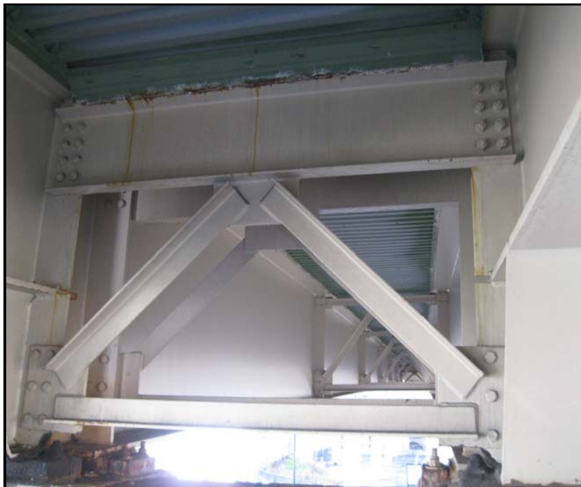
16. Rust along the top flange edge of Bay 3 diaphragm in Span 8 at Pier 7
