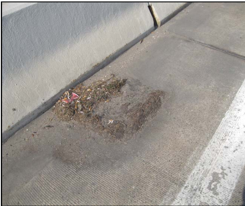
10. Clogged scupper at the NW corner of Span 2
