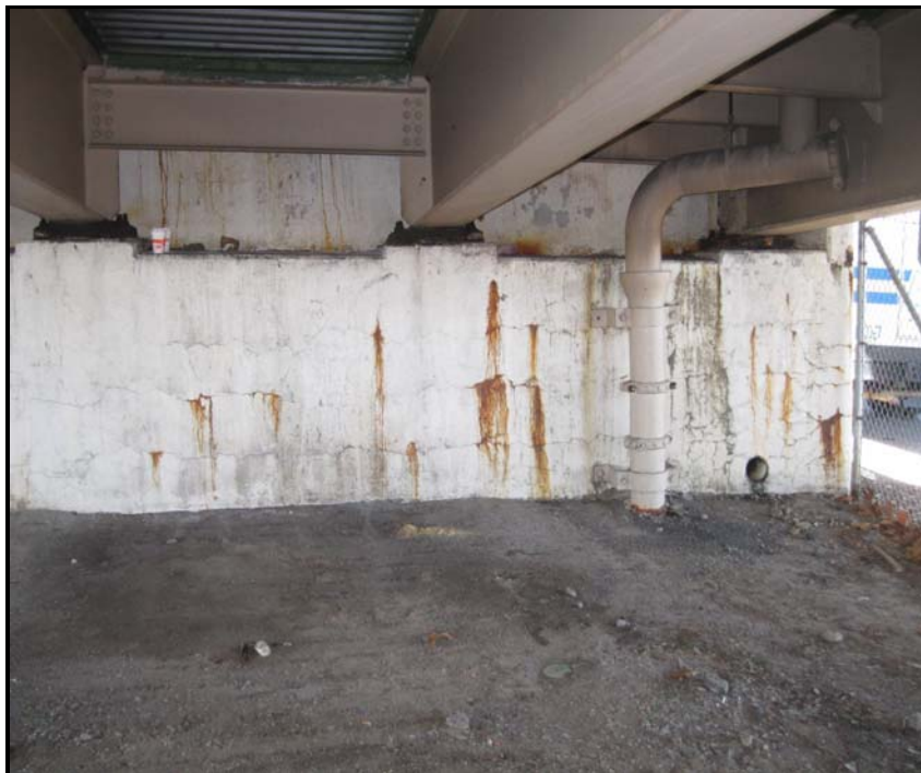
18. General view of cracks with rust in the stem of the abutment
