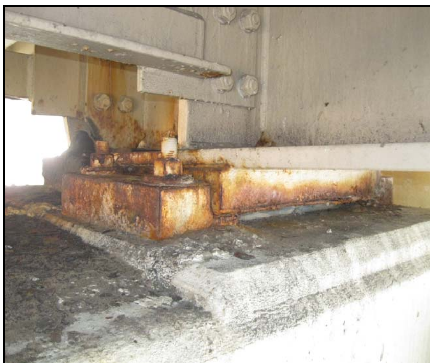
12. Rust to Bearing 4, Span 7 at Pier 7 shown
