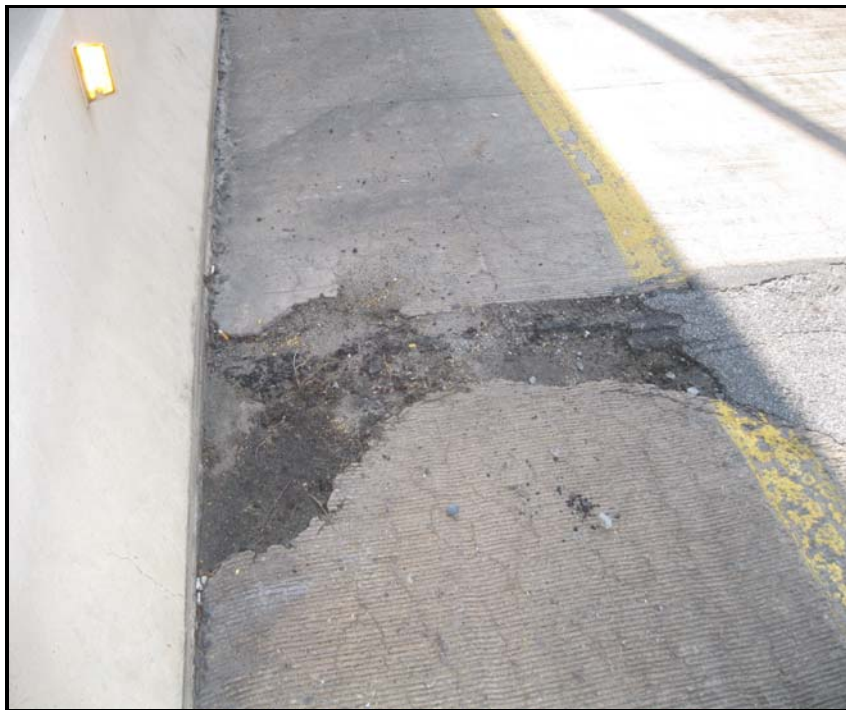
8. Spall in the North approach slab along the east shoulder
