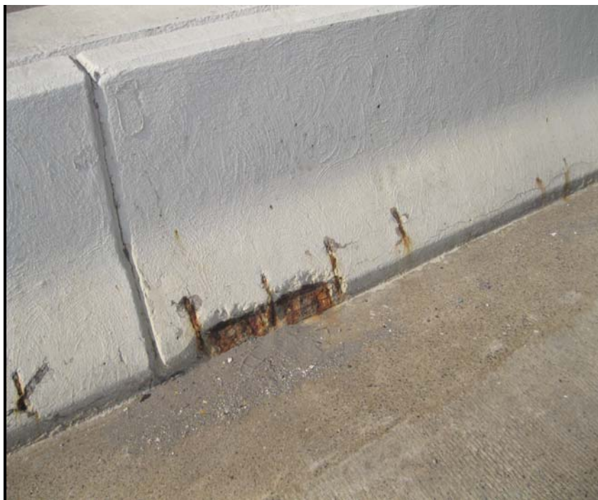
11. Spall with exposed steel at the base of the West parapet in Span 4
