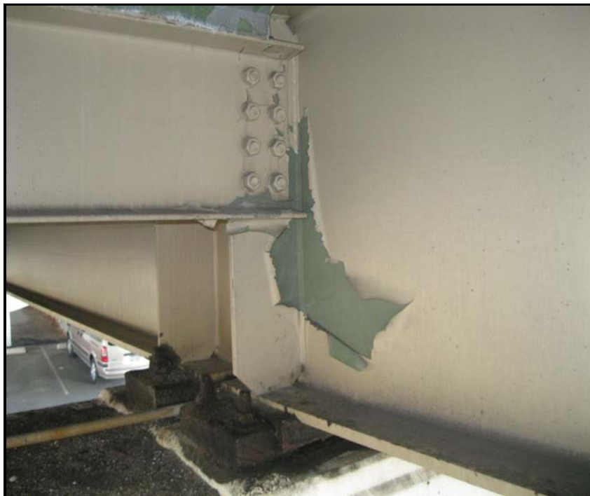
14. Peeling paint w/ exposed primer to the end of Beam 2 and Bay 2 diaphragm in Span 8 at Pier 8
