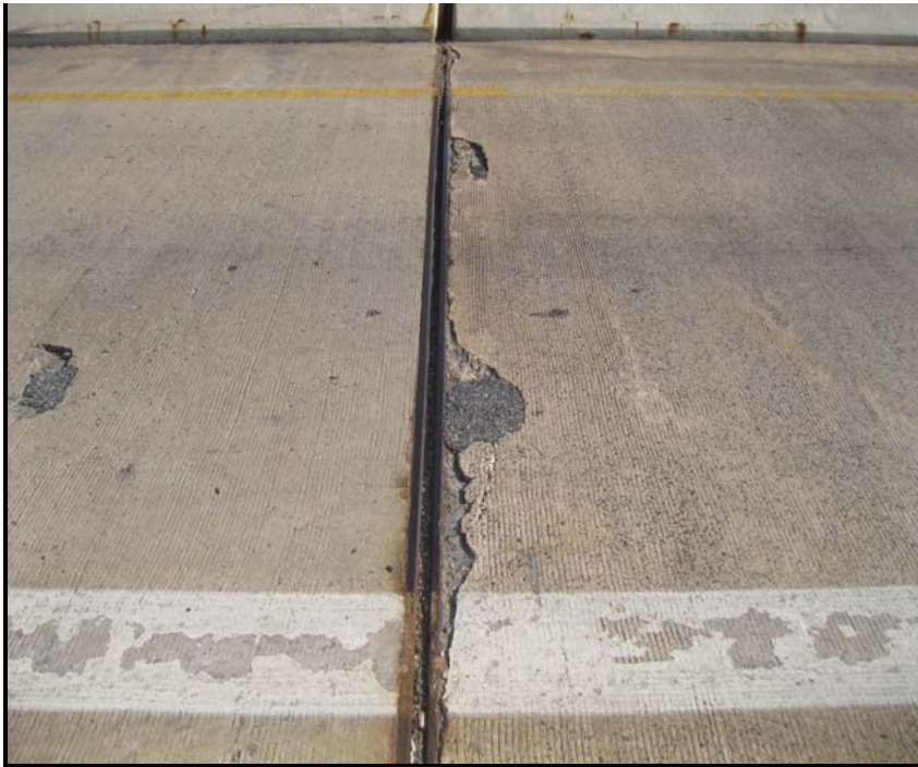
9. Spalls along the joint at Pier 4, looking East
