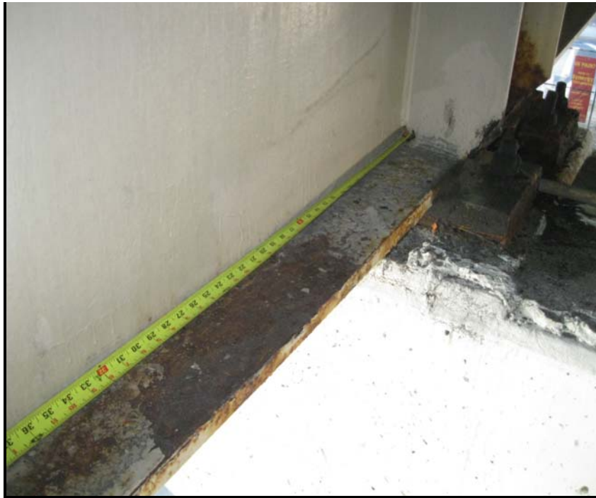
13. Rust along the bottom flange of Beam 4 in Span 9 at Pier 8
