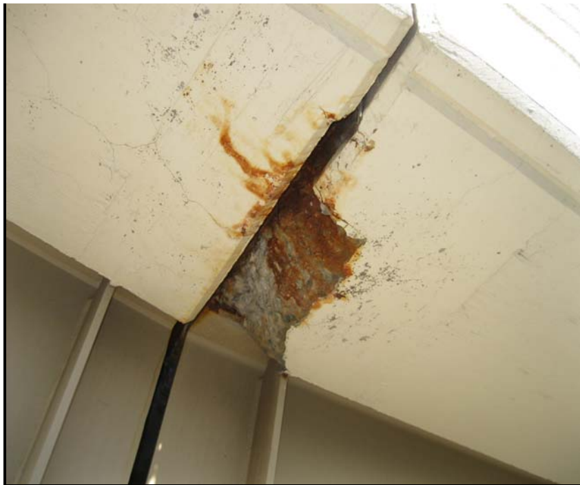
11. Typical soffit spall, South overhang at Pier 3 in Span 4
