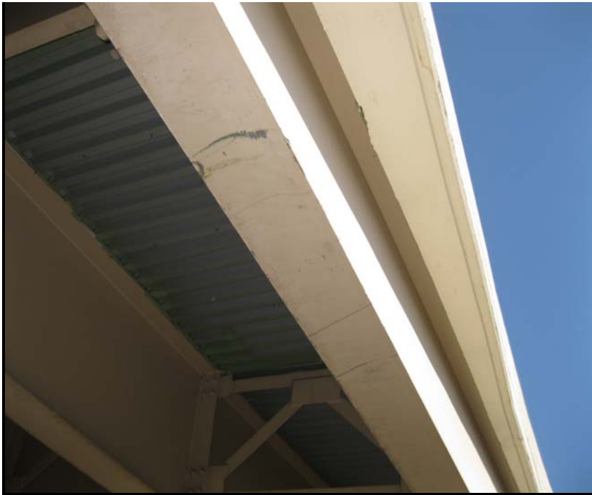
13. Scrape marks in underside of Beam 4 in Span 4
