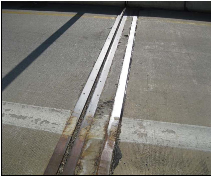
9. Spalls to the abutment header, looking Southeast
