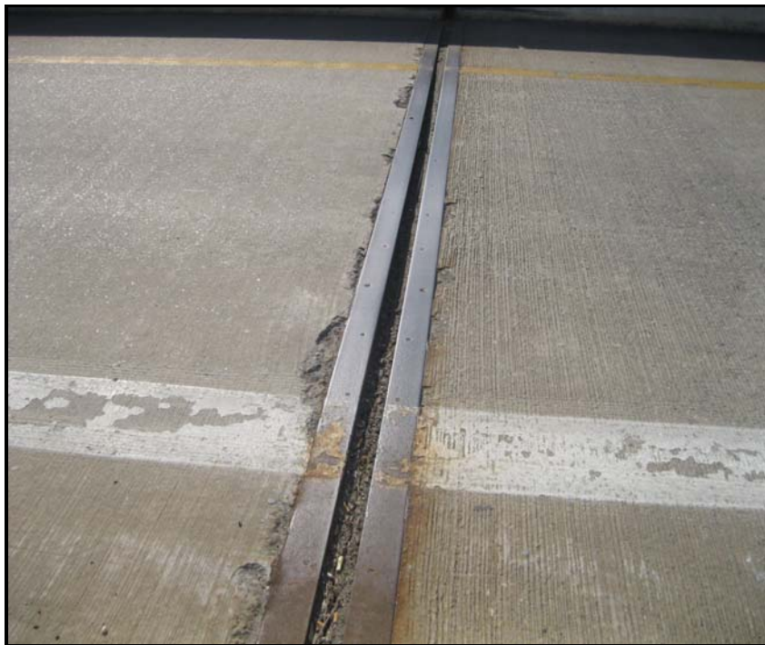
8. Typical deck joint and spalls along the adjacent deck, Pier 2, looking Southeast
