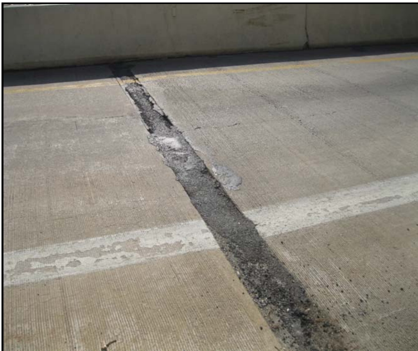
10. Deteriorated relief joint in southwest approach roadway, looking Southeast
