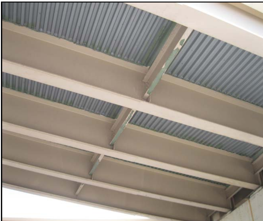
14. Peeling paint with exposed primer to the bottom flanges of diaphragms in Span 4
