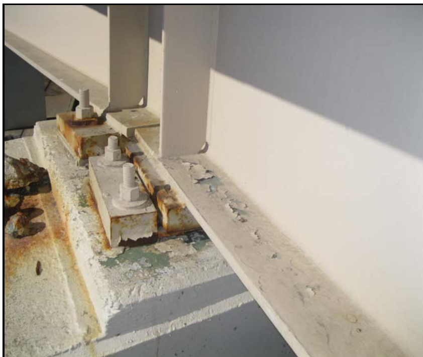
12. Peeling paint with exposed primer to the bottom flange of Beam 4, Span 4 at Pier 3
