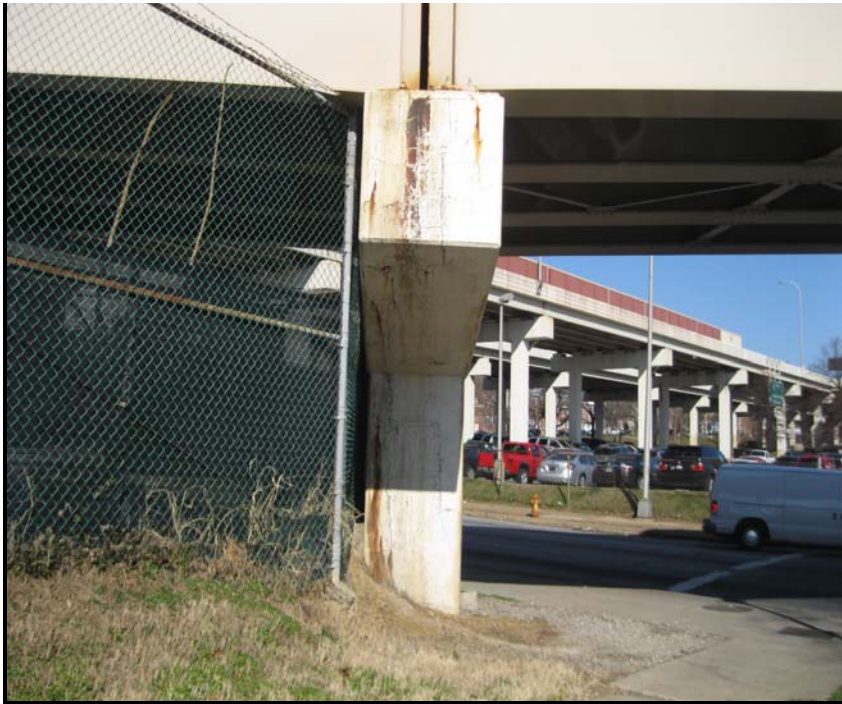
15. Cracks with rust stains in the Southeast face of Pier 1, looking North
