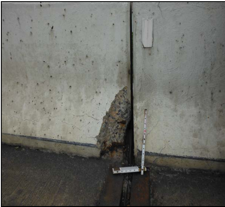
10. Span 4, N. parapet at PE9. The parapet has an 8"L x 17"H x 3"Dp spall.
