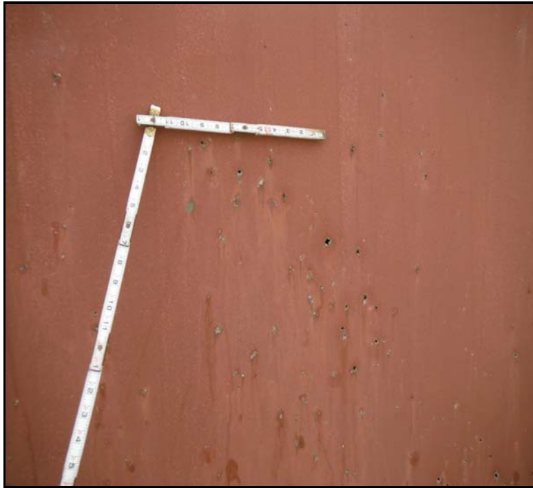
11. Span 5, N. sound wall, 4th panel from W. end. Areas of 100% SL.
