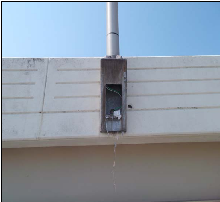
18. Span 2 light pole on N. parapet. N. side open with exposed wires and trash.
