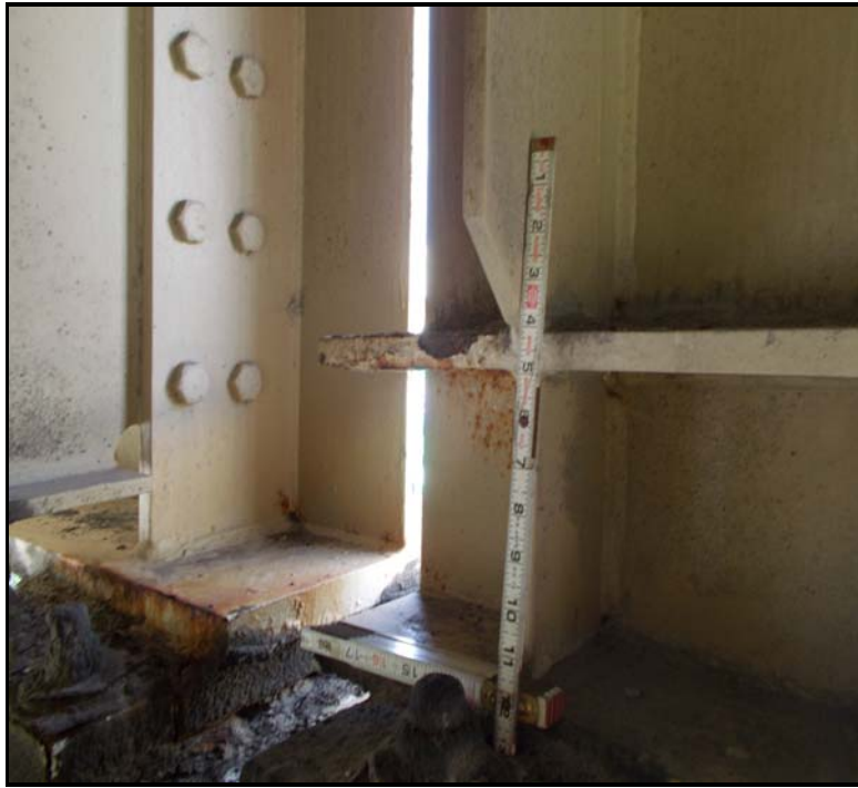
13. Span 6, BM1 at PE7 has exposed steel with surface rust.
