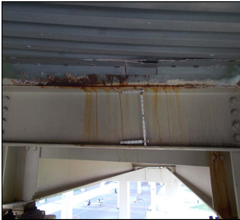
14. Span 6, Bay 1 end diaphragm at PE6 has moderate corrosion.
