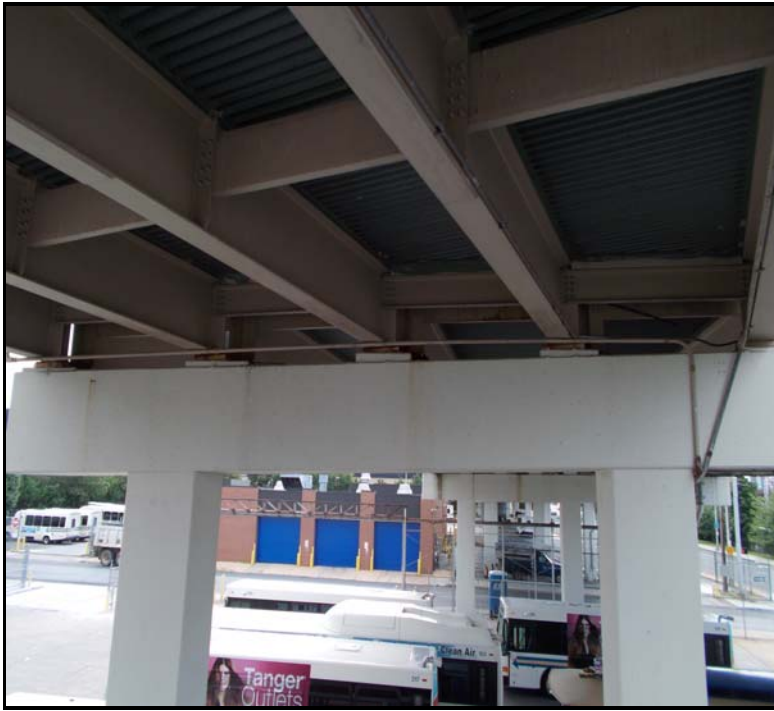
15. Span 1, PE12 has been repaired since prev. inspection (typ).
