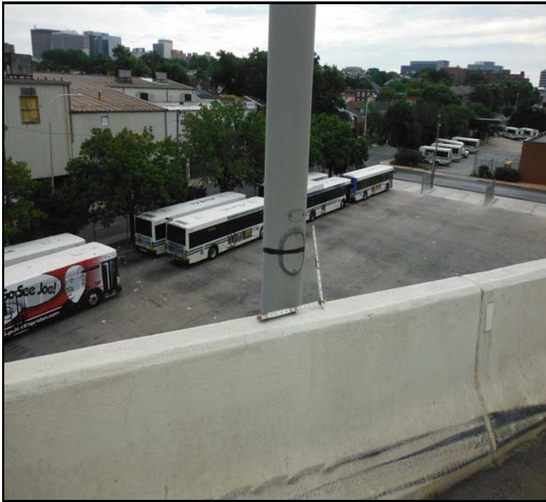
17. Span 2 light pole handhole cover has been replaced since prev. inspection.
