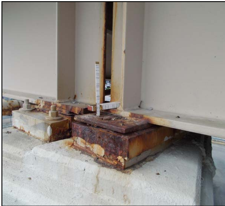
12. Span 1, Brg 5 @ PE12. N. AB sheared off and pack rust btwn plates.
