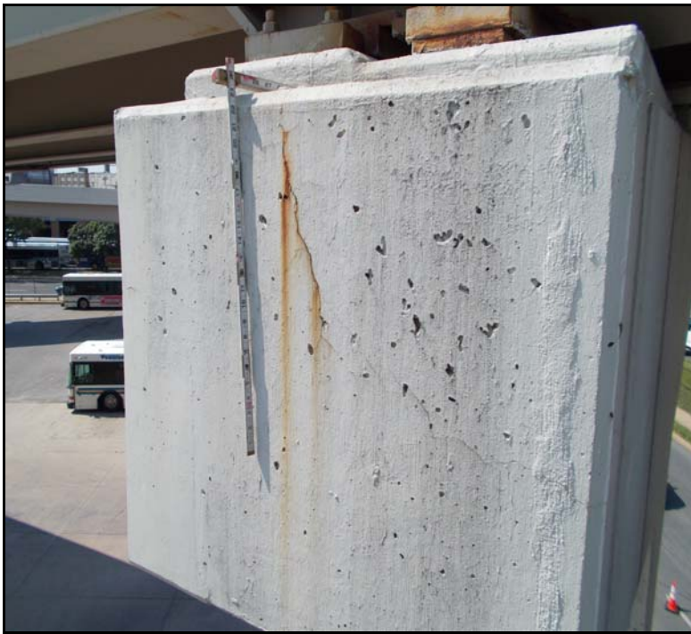
16. PE8, N. end of cap has a crack with corrosion staining.
