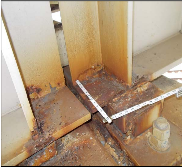
17. Span 2, G1 at P02A - Previously painted S.L. w/ exposed steel in web and flg.
