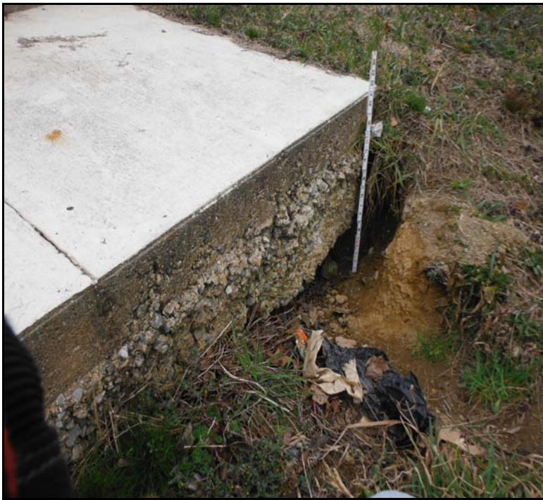
22. NE Wingwall at NE corner - 54" L x 24" W x 22" D area of erosion.
