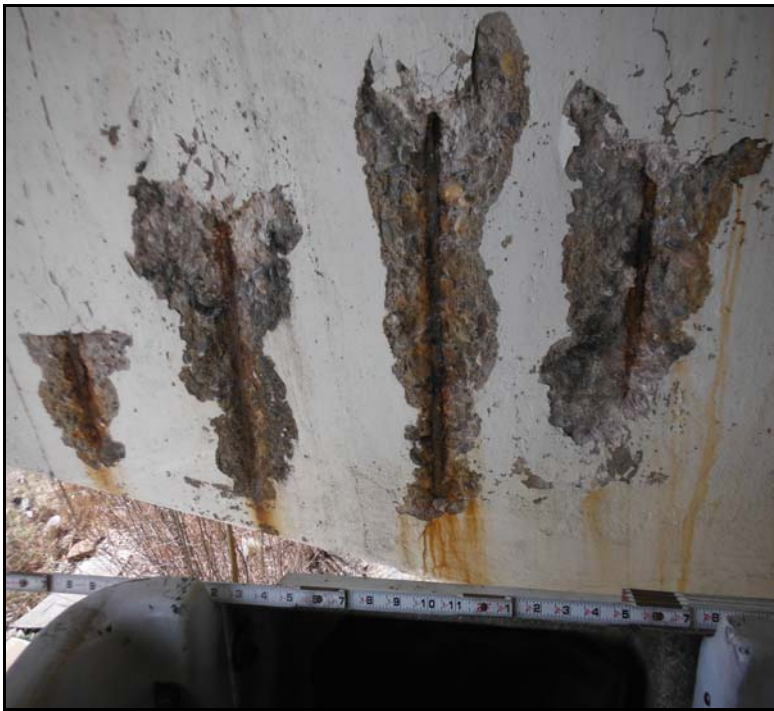
20. Pier 3A, N face @ Bay 3 - 42"W x 24"H area w/ 4 spalls w/ exp corr steel reinf.
