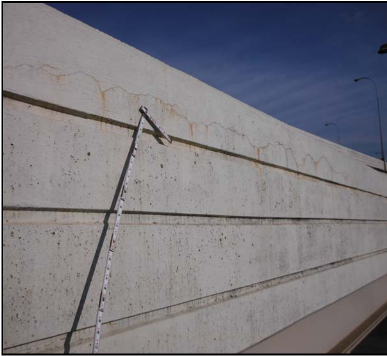
15. Span 4, E Ppt exterior face@ midspan - 10' L x HL crack w/ minor rust staining.
