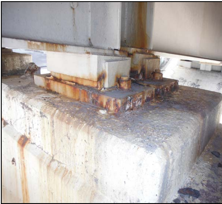
18. Pier 5A, BM 4, Span 5 Brg - Flaking paint w/ corrosion and rust lam on plates.
