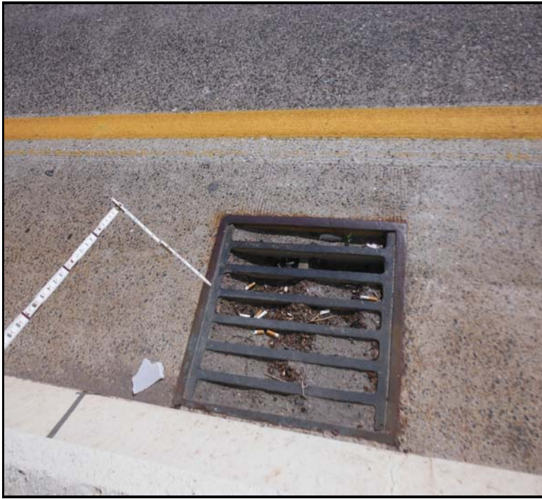
11. Span 4, W shoulder - Clogged scupper.
