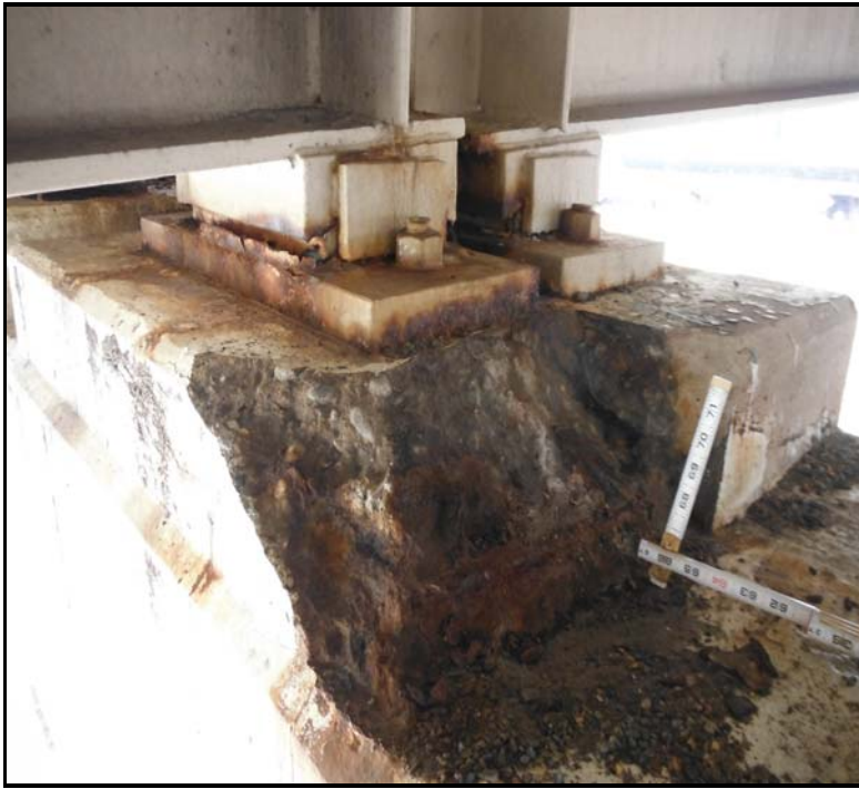
19. P05A, Ped 4, SW corner - 12"L x 18"W x FH spall w/ exp corr steel reinf.
