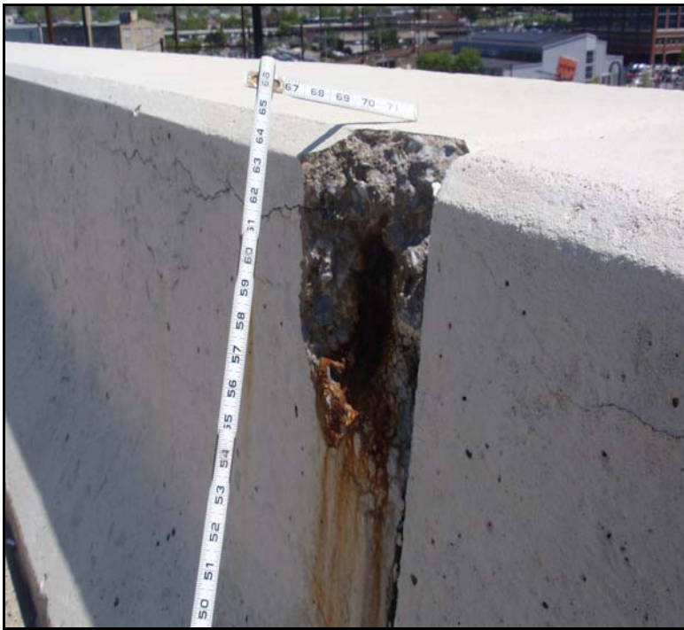
14. Span 1, E Ppt at S end - 7"L x 11"H x 3"D spall @ top w/ exp corr steel reinf.
