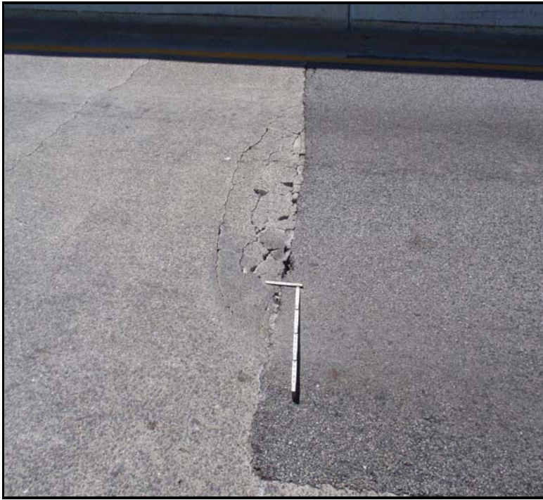
9. Span 5, S of bitum patch - 1/4" W cracks & up to 2" Diam x 1 1/2" D spalls.
