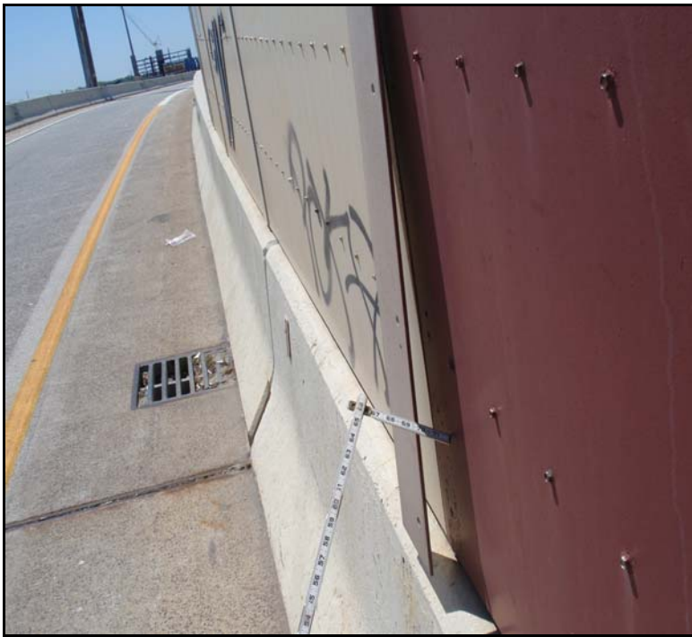
16. Span 2, W Ppt steel railing @ S end - Splice panel missing 6 of 8 fasteners.
