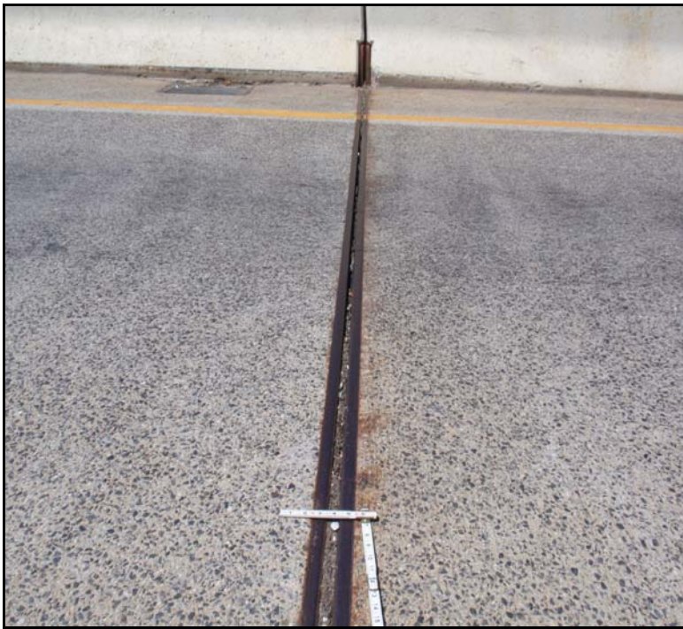
12. Pier 1A deck joint - Debris full-width and minor tears throughout.
