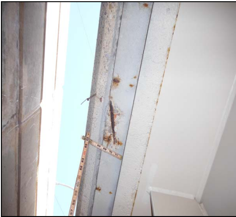
10. Span 1, N o/hang at midspan - 6"L x 3"W x 1 1/2"D spall w/ exp corr steel reinf.
