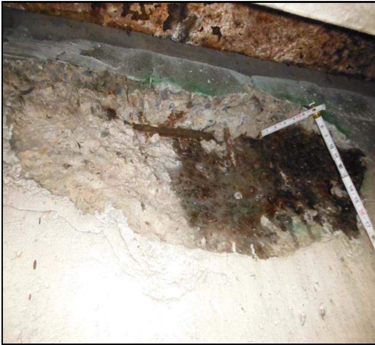
21. N Abut backwall @ Bay 3 - 15" H x 32" W x 3" D spall w/ exp corr steel reinf.
