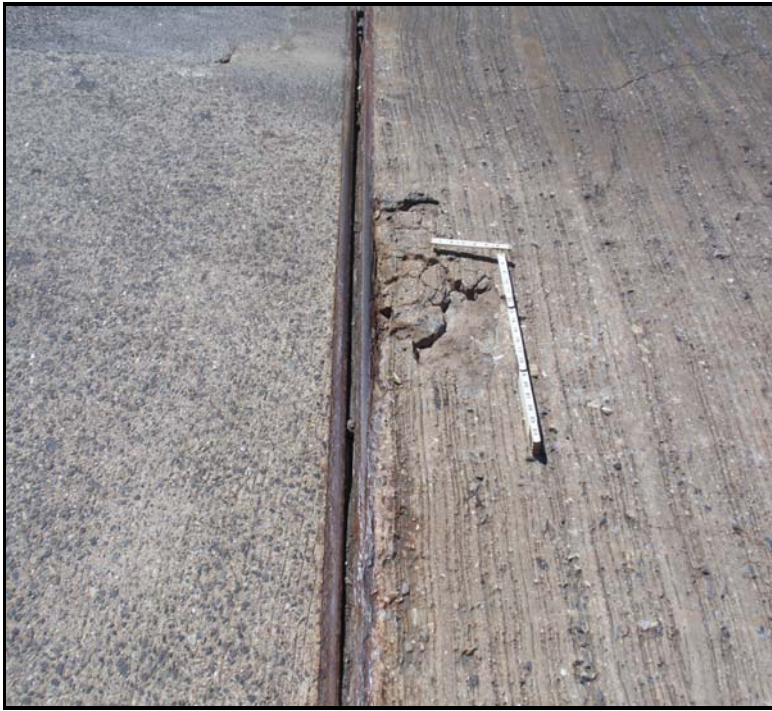
13. N Aprpr slab - 22" W x 11" L x 1" D spall & adj. joint armoring w/scrapes.
