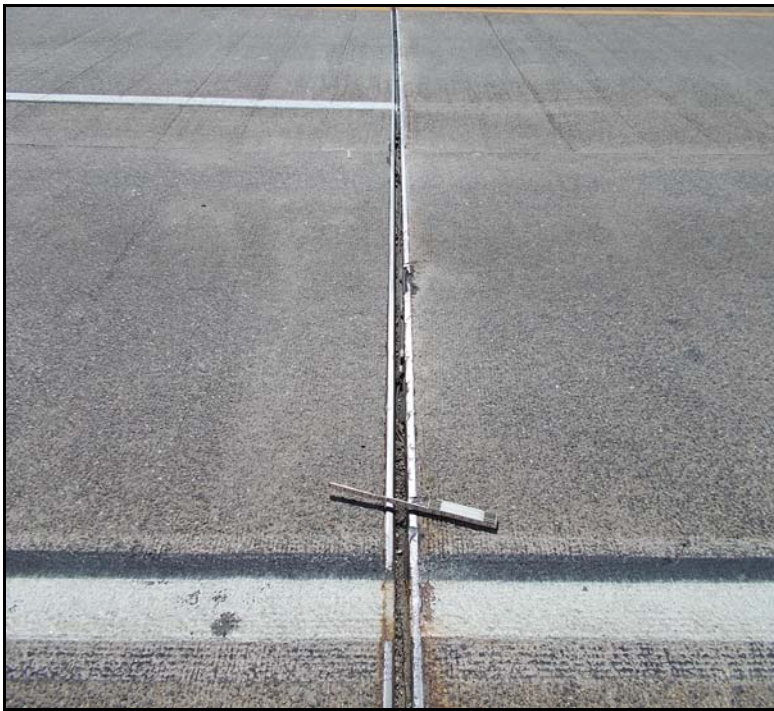
18. Span 55, right lane is missing extrusion.
