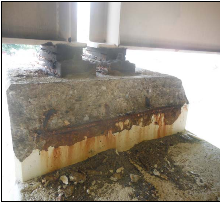
22. Span 41, Pedestal 1 east face with spall with exposed steel.
