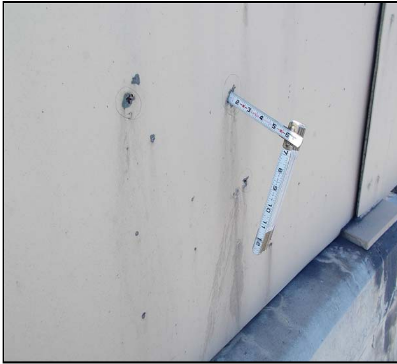
19. Span 28, W. Parapet barrier with holes.
