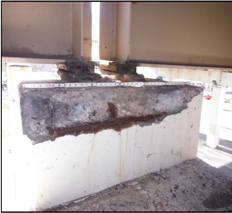
25. Span 54, Pedestal 6 spall with exposed steel.
