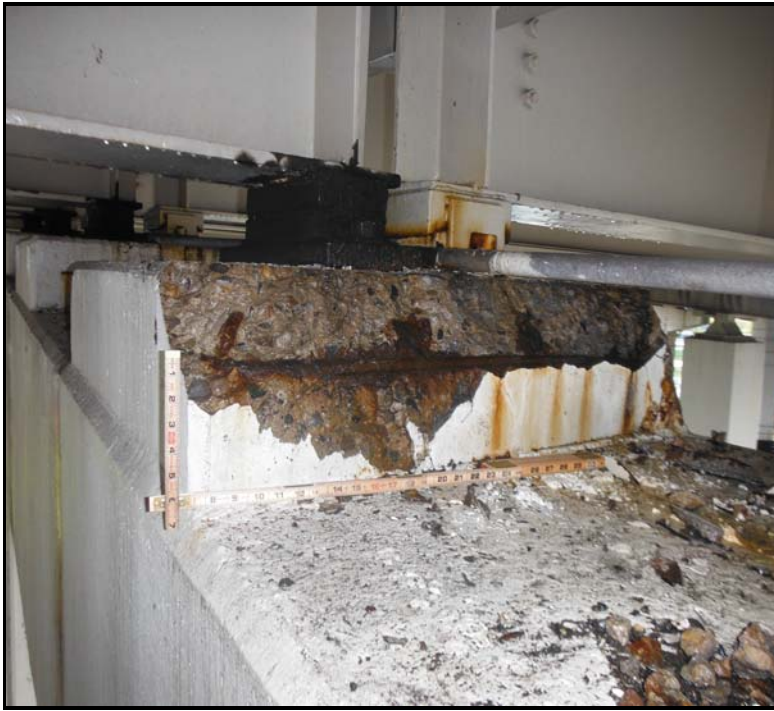
21. Span 27, Pedestal 4 west face with spall with exposed steel.
