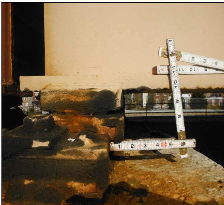
23. Span 44, Brg 6 at Pier 43, overcontracted at 65 deg.
