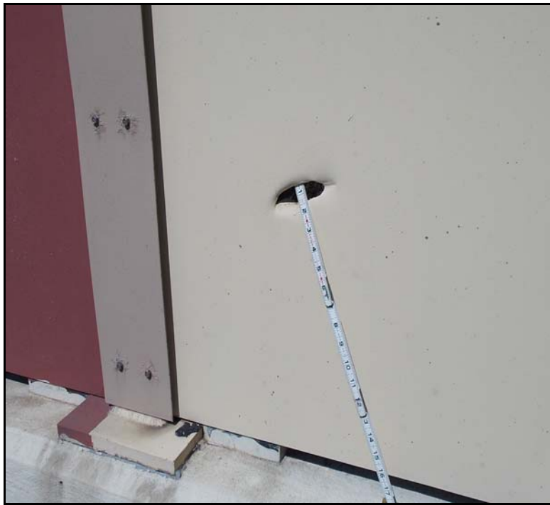
20. Span 52, Panel 5 of metal rail has a hole.
