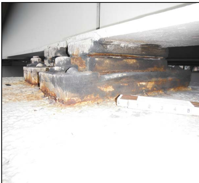
24. Span 52, Brg 6 at Pier 51. NE corner w/ pack rust (appears frozen).
