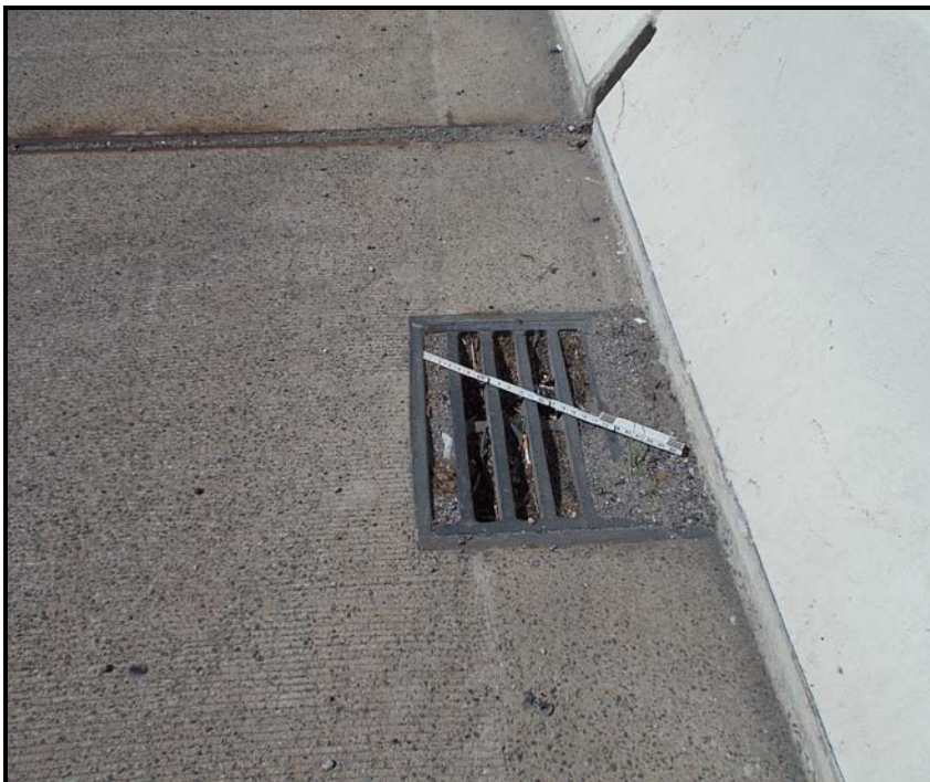
22. Span 27, East Shoulder - Typical clogged scupper.
