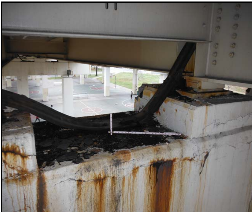
24. Pier 55 joint u/s - Joint material hanging down onto Pier 55 cap.
