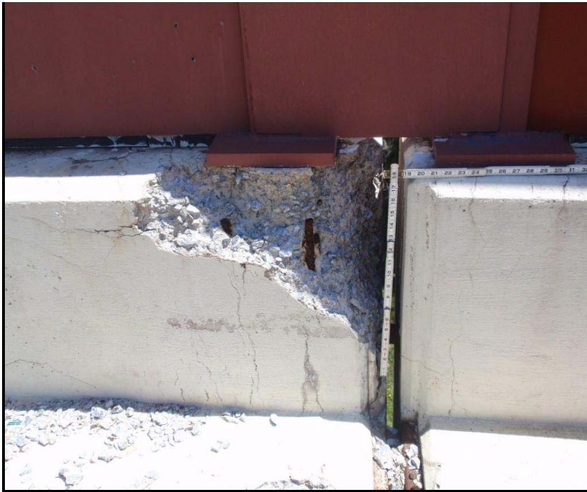
25. Sp 59, East Ppt - 20" L x 14" H x 10" D spall w/ exp corr steel reinf.
