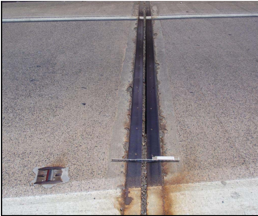
23. Pier 52 strip seal joint - Typ debris, depressed & debonded material.
