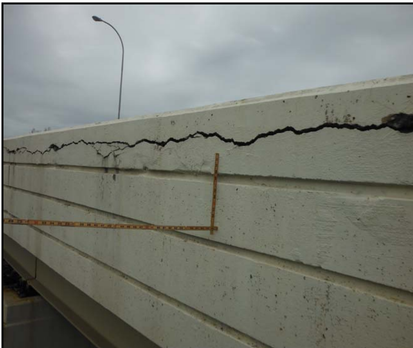
26. Span 46, W. Ppt ext face, n. end - Up to 5/8" W horizontal crack.
