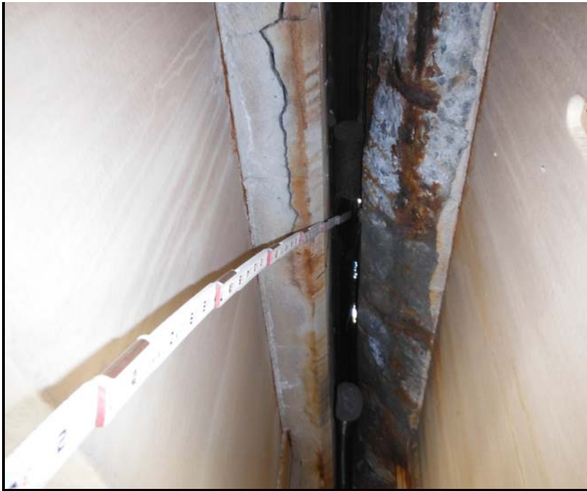
21. Span 54, Bay 3 n. haunch - 7' L x FW x 4" D spall w/ exp corr steel reinf.
