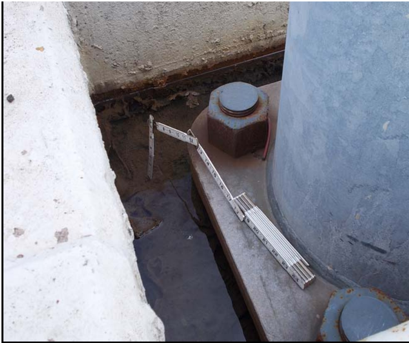
29. Sp 43, E. Ppt conc box for sign struct. - Ponding water up to 3 1/2" D.
