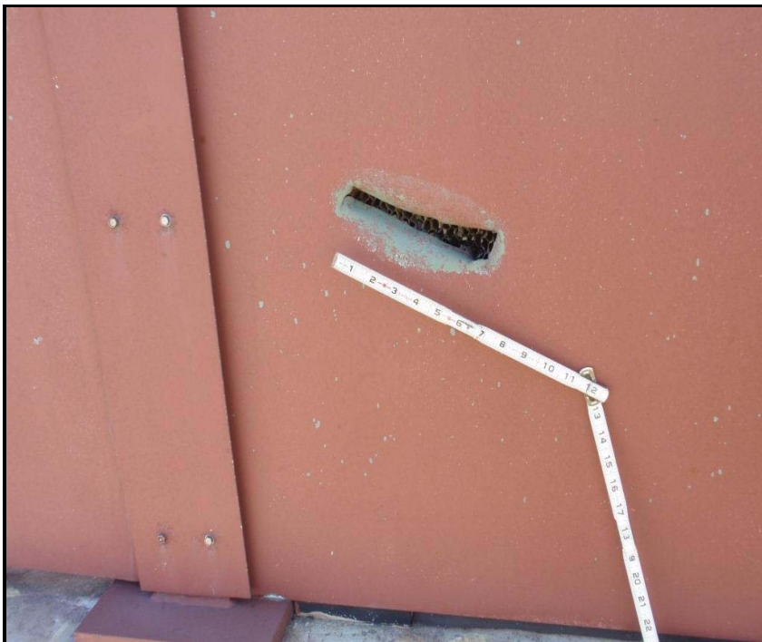
30. Sp 46, E. Ppt metal railing - 6 1/2" L x 1 1/2" H hole in panel.
