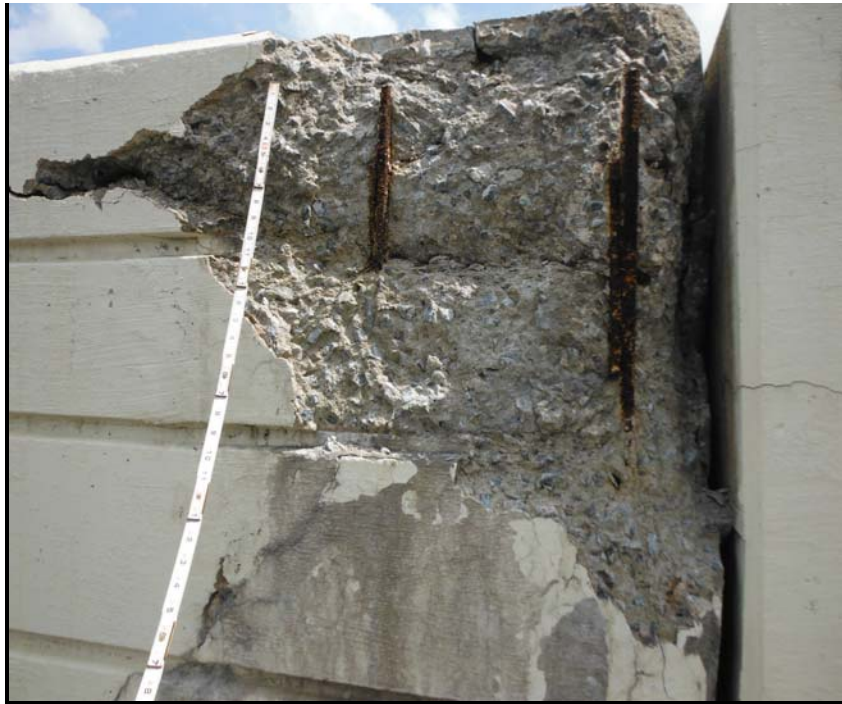
27. Sp 56, W. Ppt ext face, s. end - 3' L x FH x 4" D spall w/ exp corr steel reinf.
