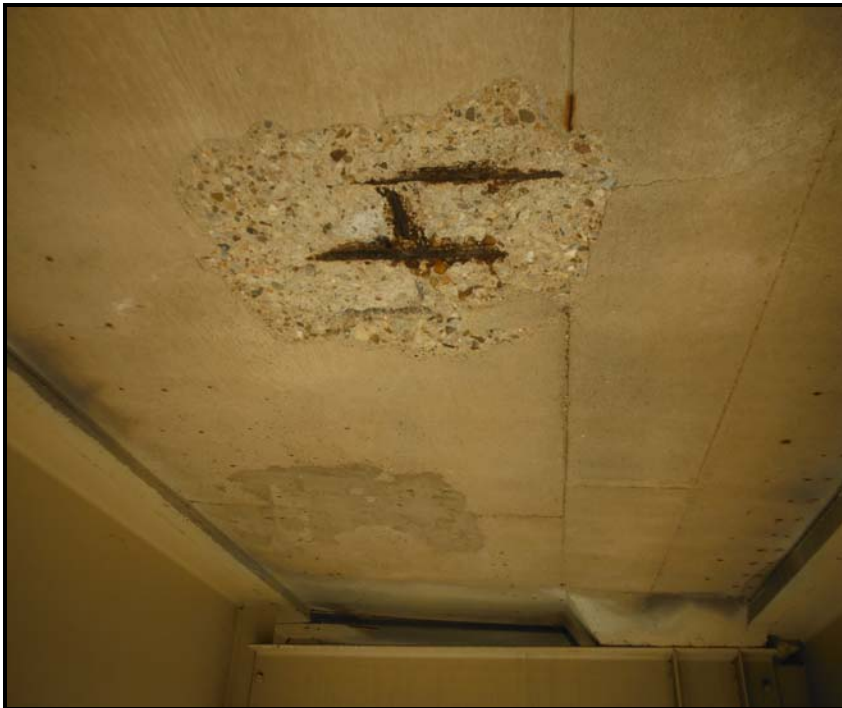
20. Span 42, Bay 5 at N. end - 26" L x 22" W x 2" D spall w/ exp corr steel reinf.
