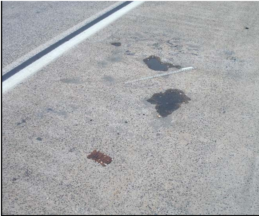
19. Span 32, East Shoulder, looking north - Fire damage.
