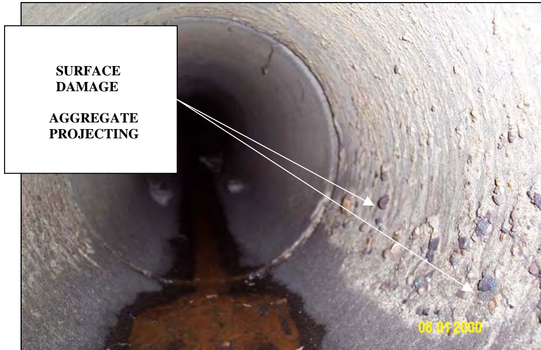
Fine material eaten away showing complete aggregate.
