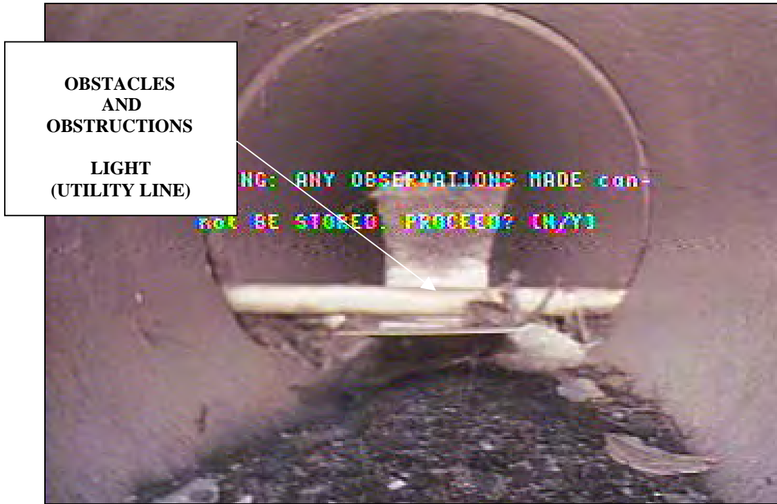
Obstruction blocking hydraulic capacity – Utility Pipe
