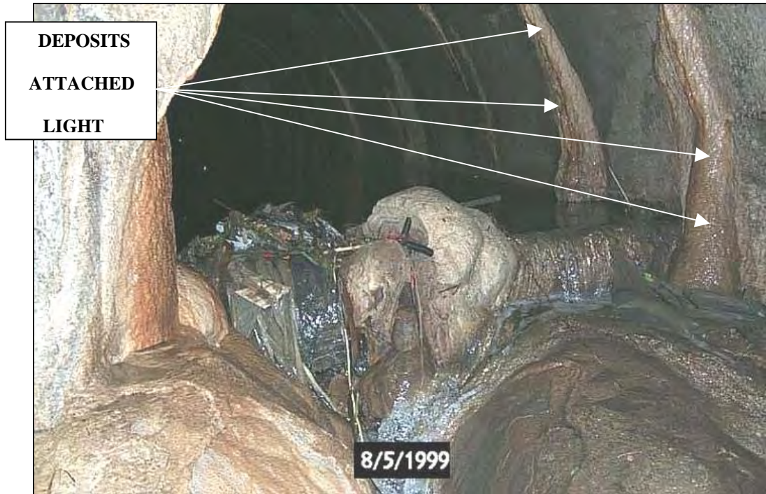
Accumulated materials block less than 40% of pipe diameter.
