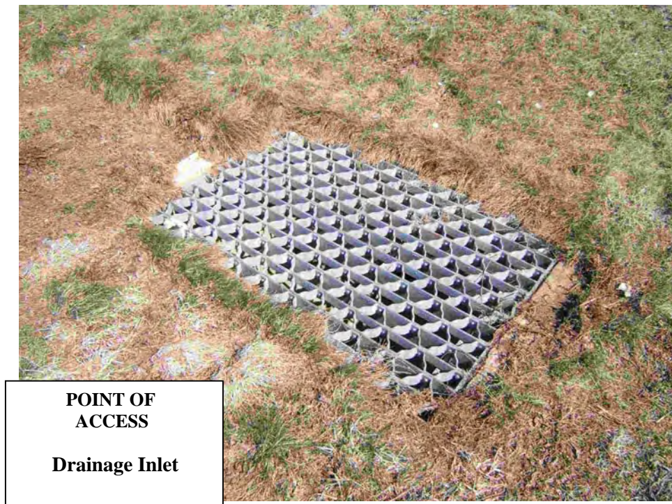
Parkway Drainage Inlet.
