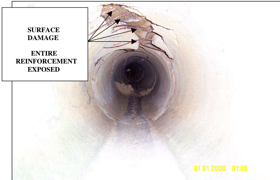
Wall material loss exposing entire reinforcement.
