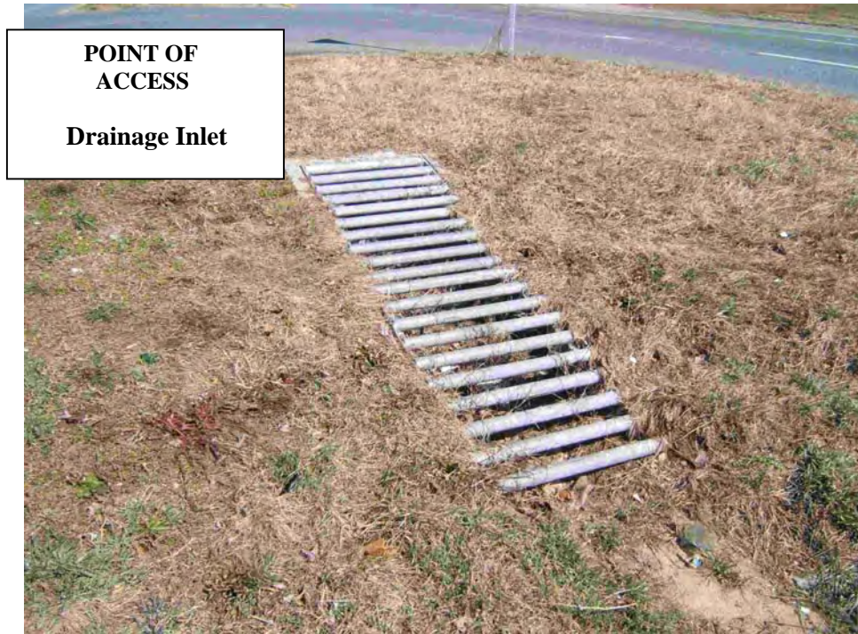
Safety End Drainage Structure.
