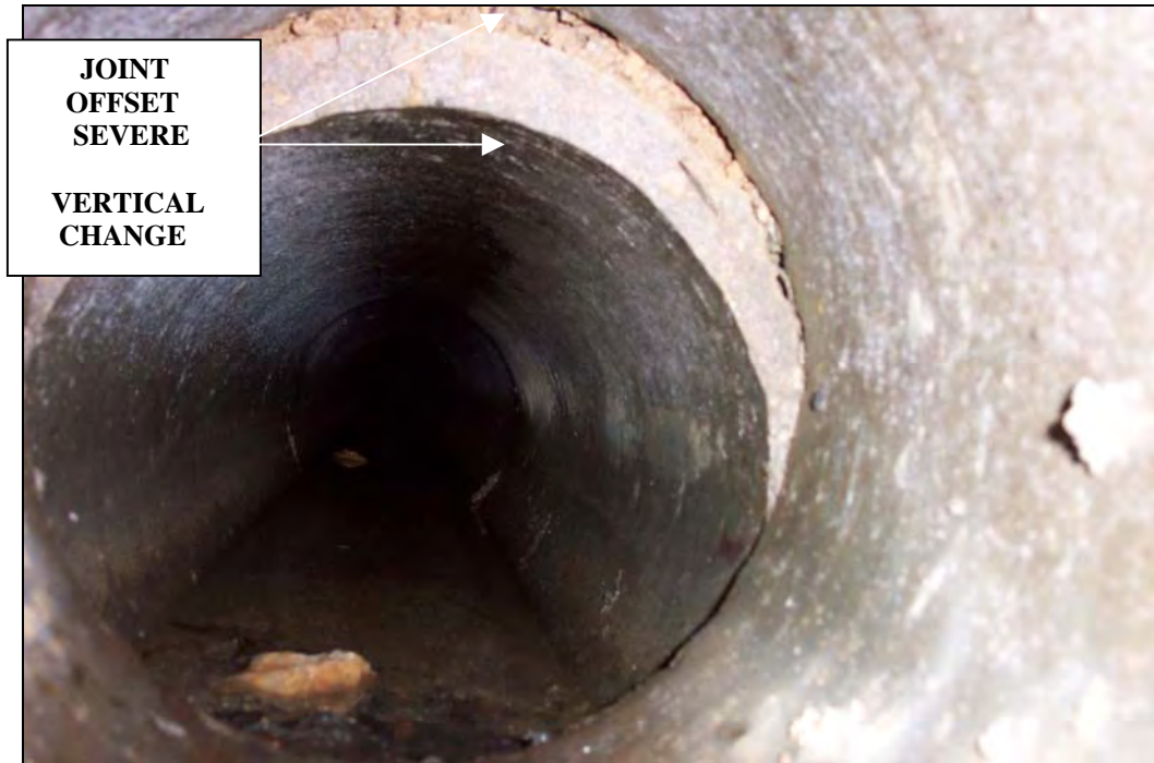
Joint level-shifts – no joint match.
