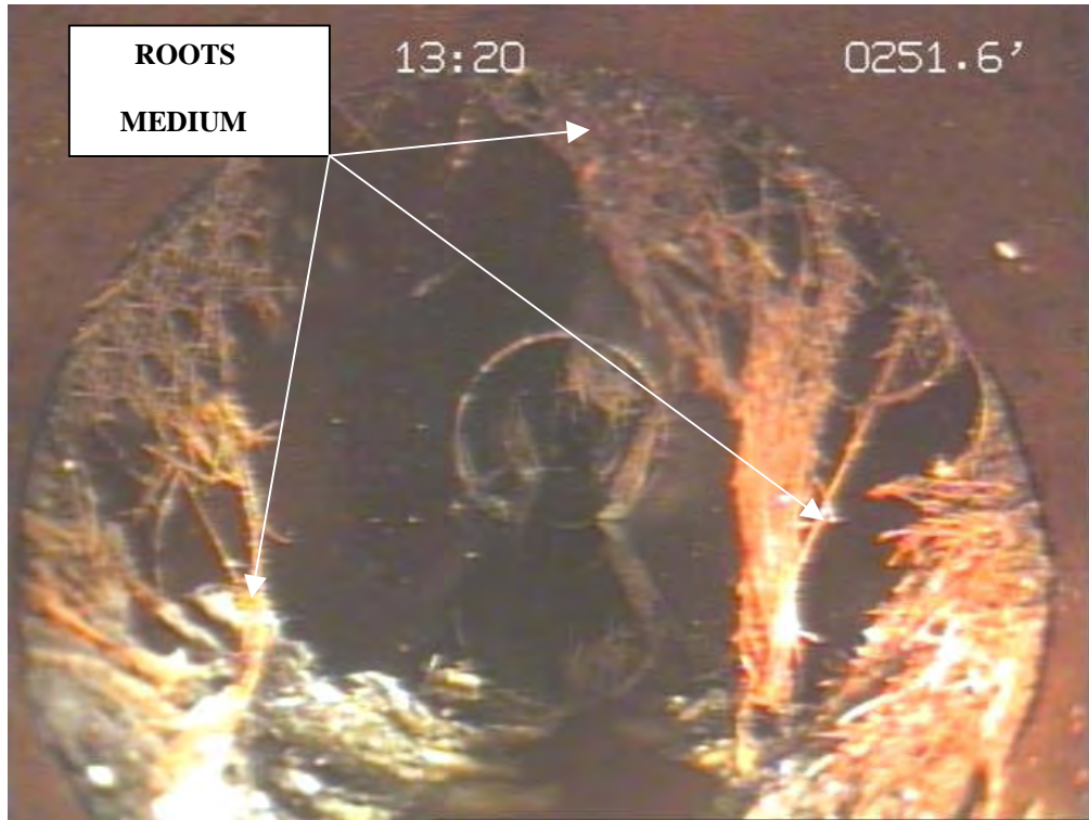
Root growth less than 50% of pipe.
