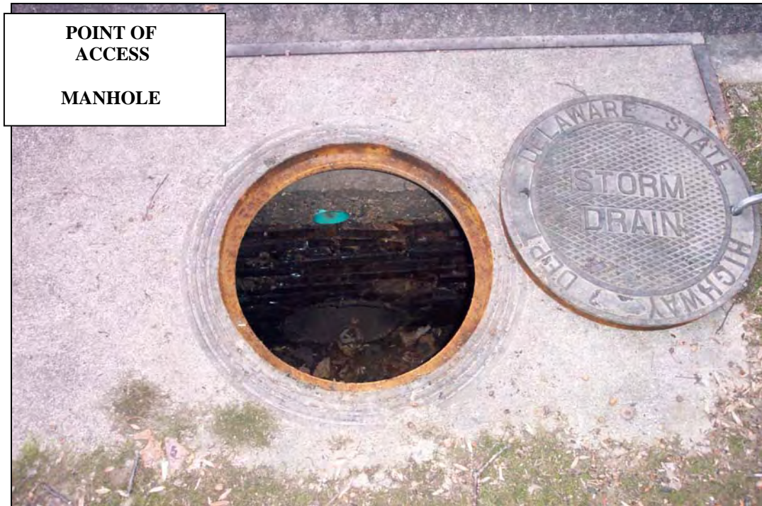
Manhole access to storm sewer system.
