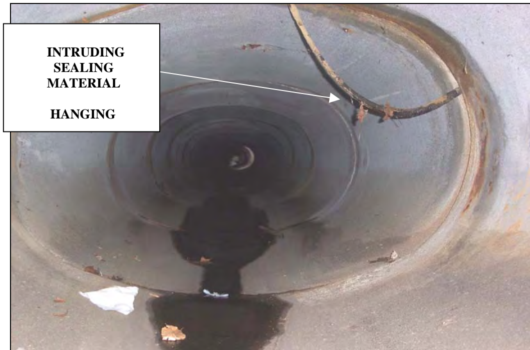
Joint seal material hanging inside pipe
