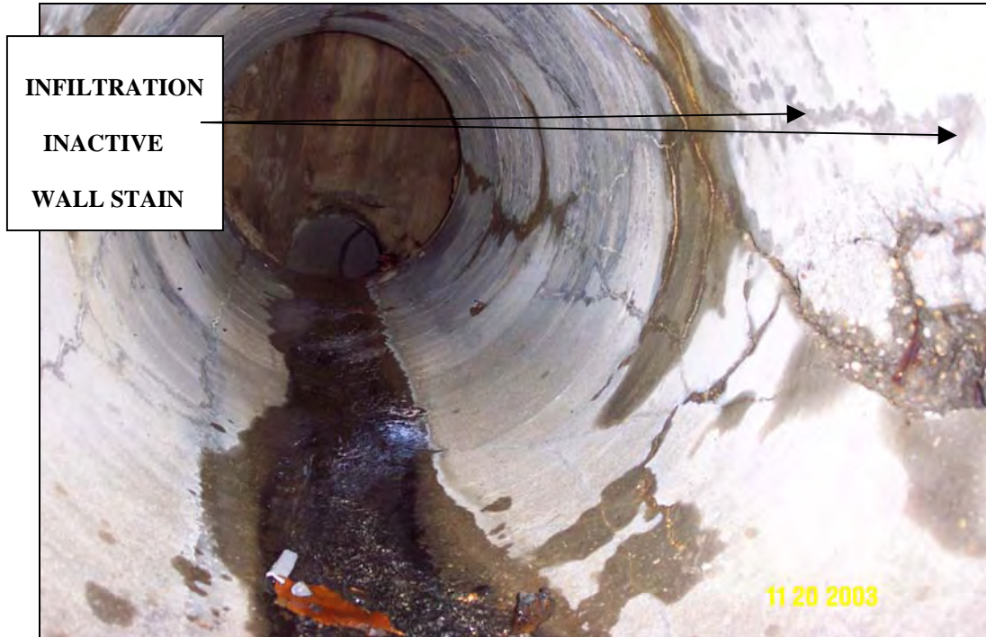
Past leak evidenced by stain on wall.
