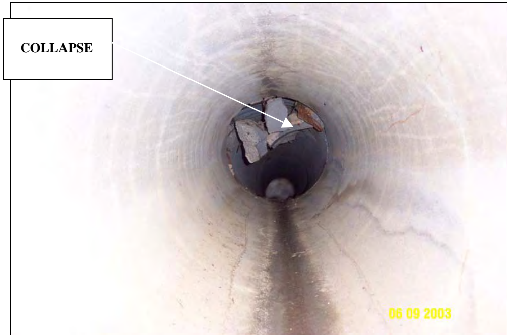
Collapse - of RCP
