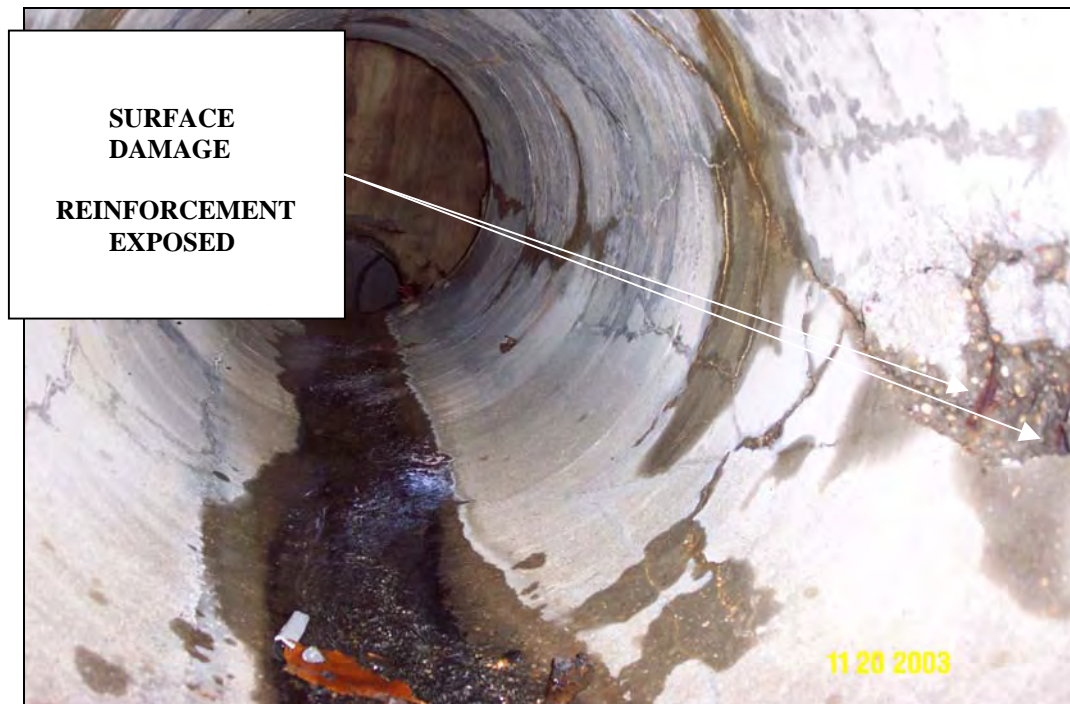
Wall material loss exposing reinforcement surface.
