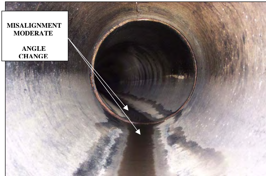
Pipe changes direction at a joint causing gap on side(s).
