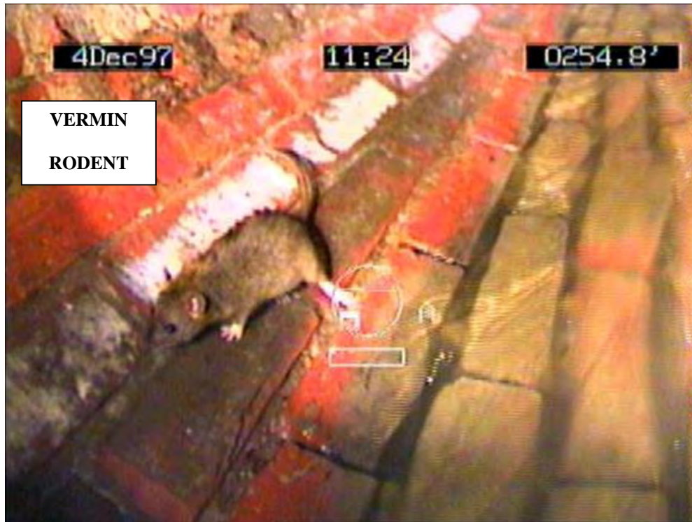
Vermin (Rodent) in pipe
