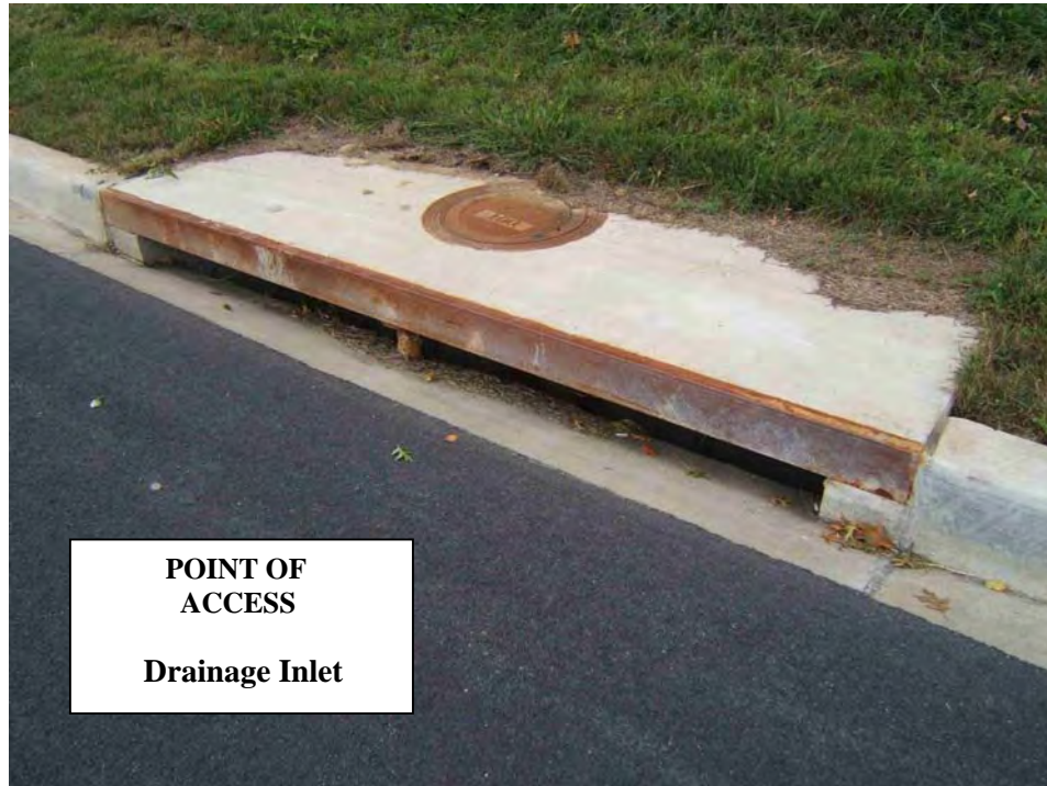
Curb Opening Drainage Inlet.
