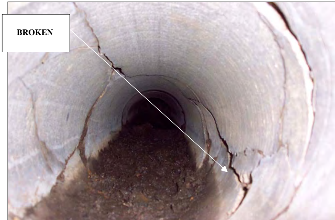
Visible displacement of pipe/structure material from its original position
