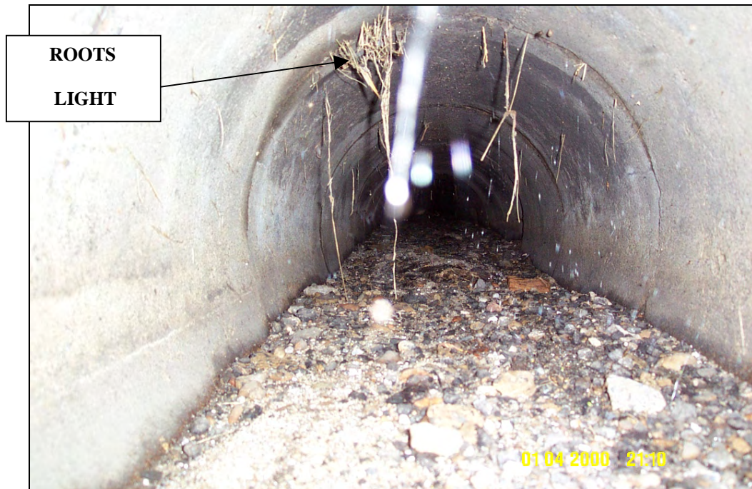
Light root encroachment into pipe.
