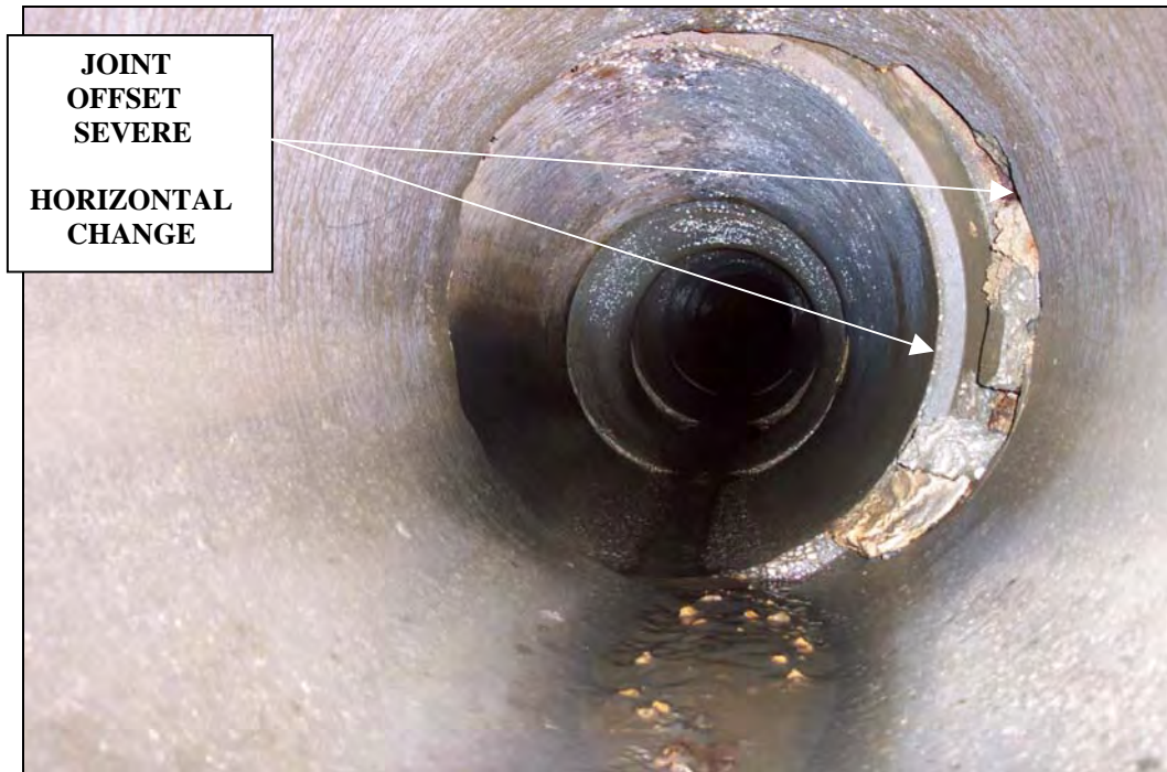
Joint side-shifts – no joint match.
