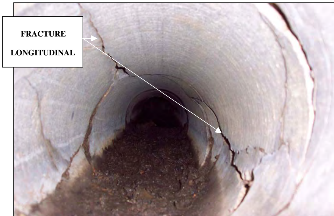
Fracture runs along the axis of the pipe (parallel to the centerline).
