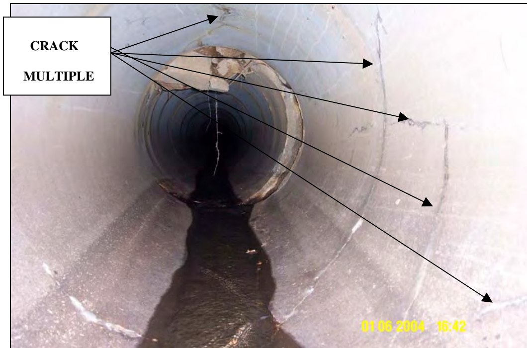
Combination of circular, longitudinal, and/or spiral cracks
