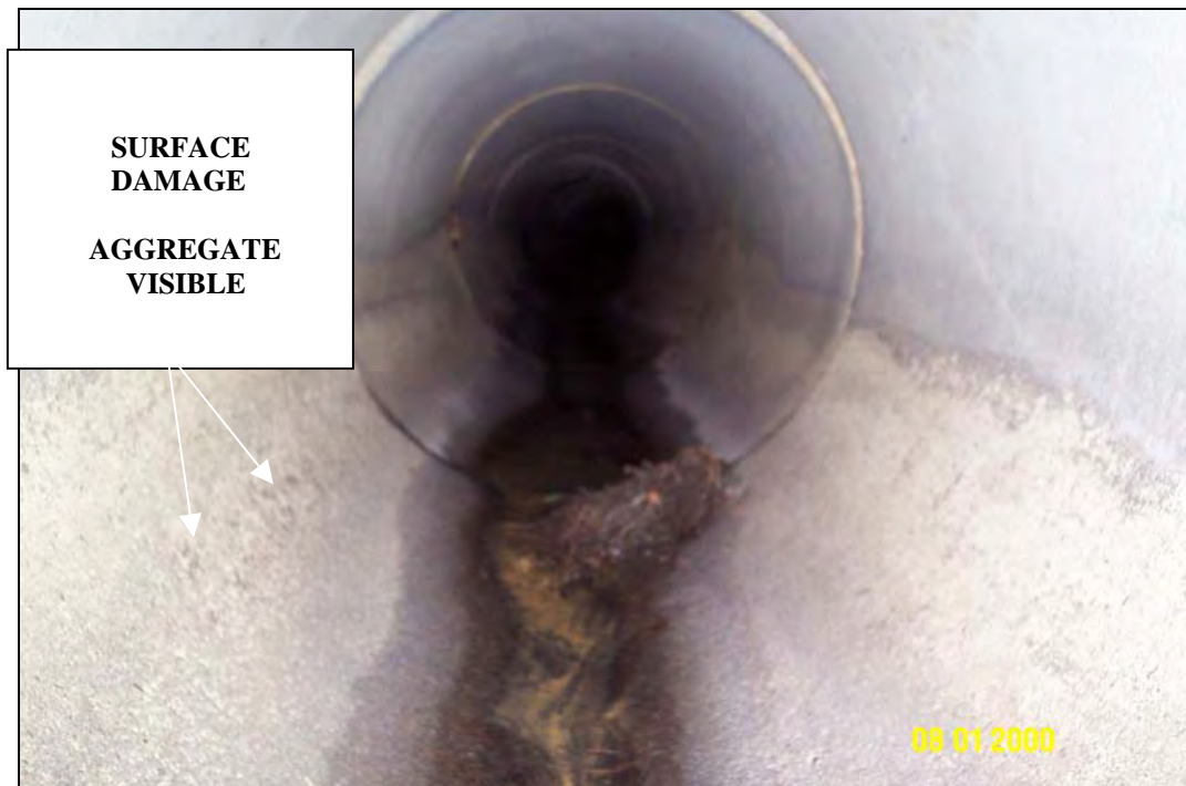
Fine material eaten away showing aggregate surface.
