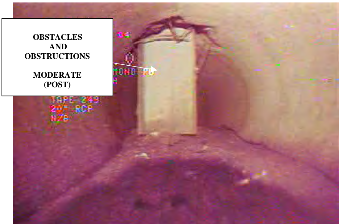
Obstruction blocking hydraulic capacity – Guardrail Post
