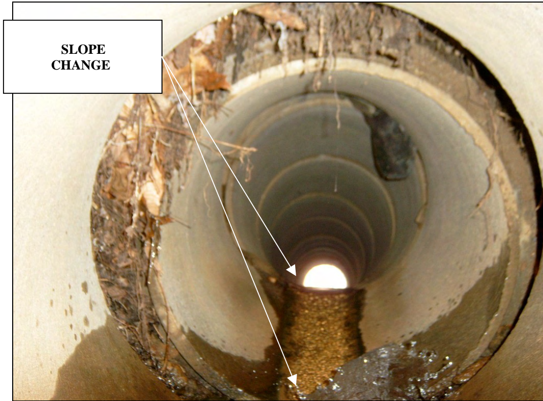
Connected pipe sections change elevation up or down.
