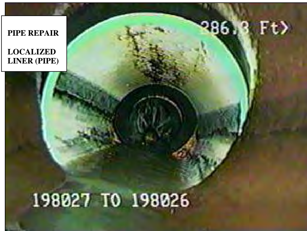
Original pipe section(s) repaired using localized liner.
