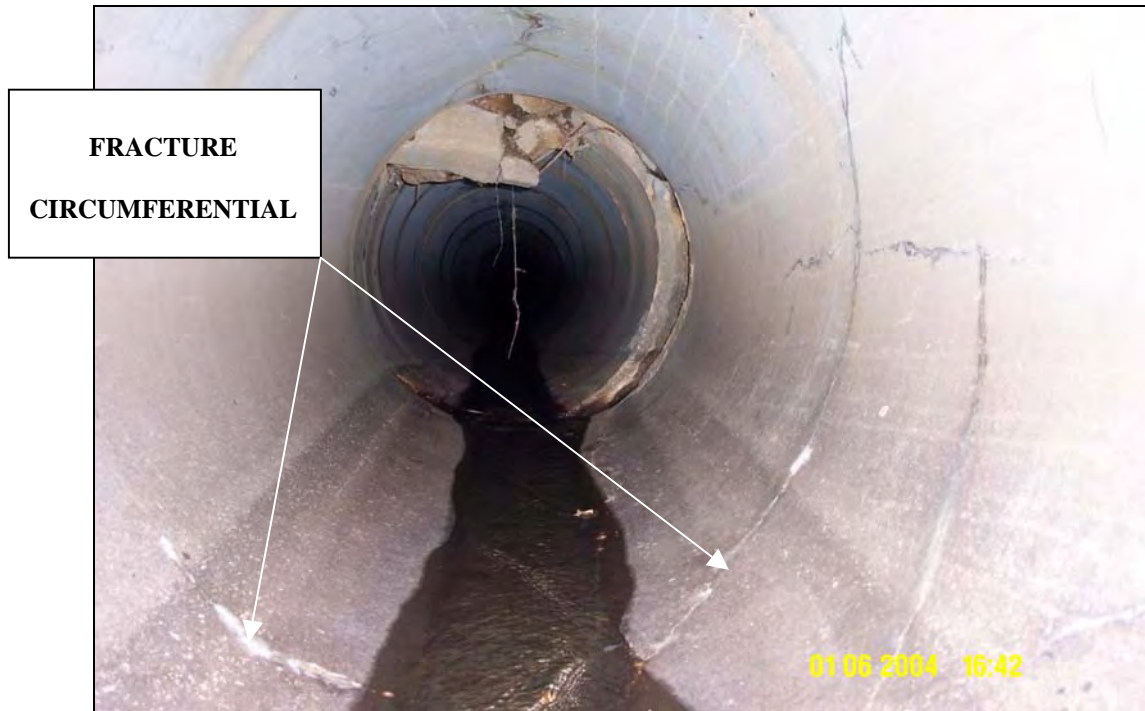
Fracture runs at right angles to the axis (parallel to the joints).
