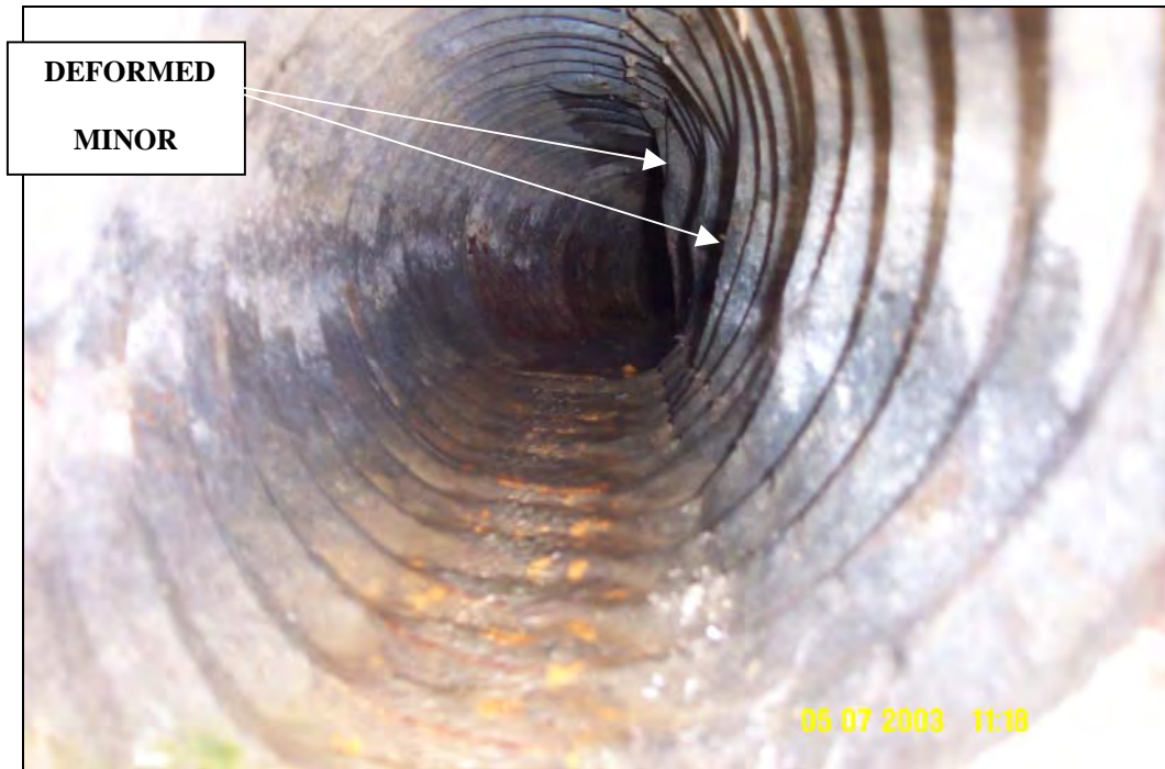
Slight alteration to original cross section.
