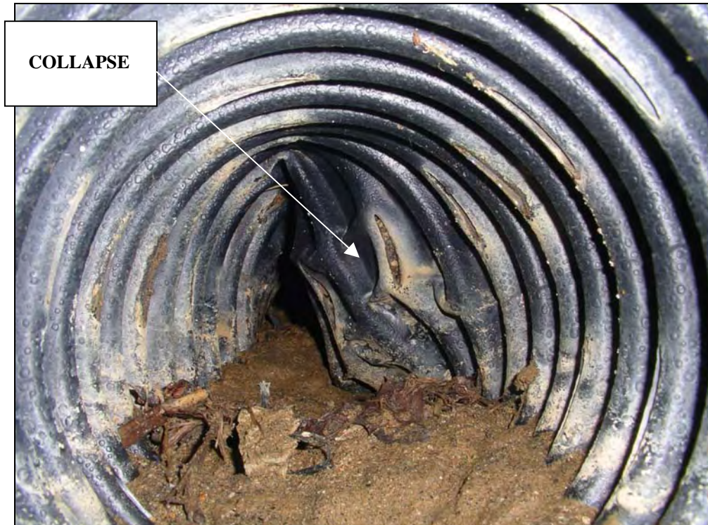
Collapse - of CMP
