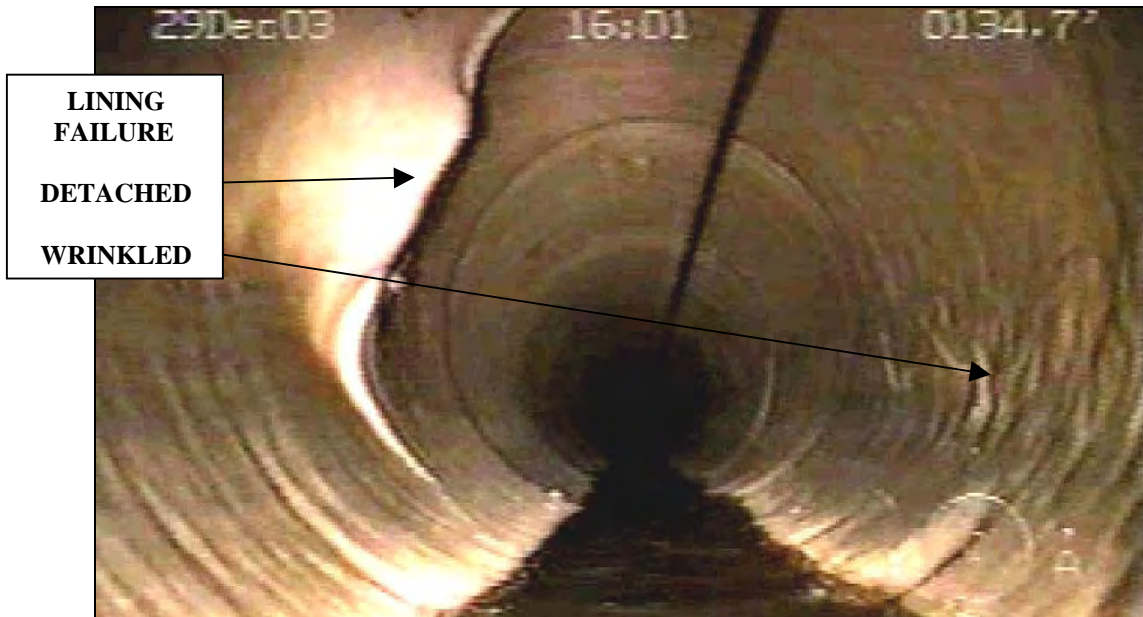
Lining no longer formed to original cross surface - Wrinkled (not smooth) Defective Surface
