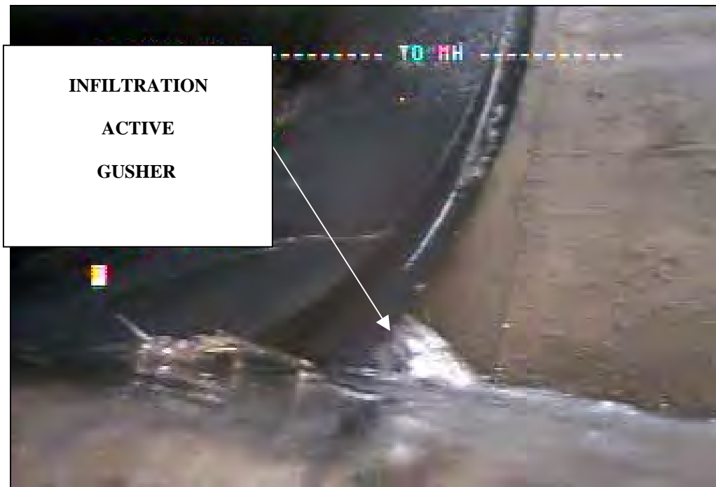
Gushing water infiltration.
