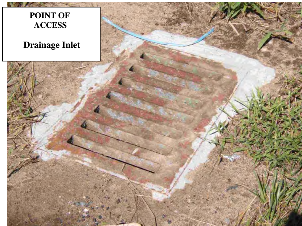
Lawn Drainage Inlet.
