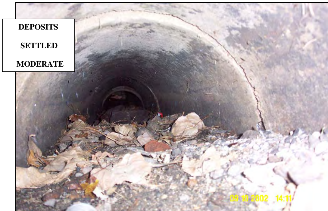
Accumulated materials blocking 20-40% of pipe diameter.
