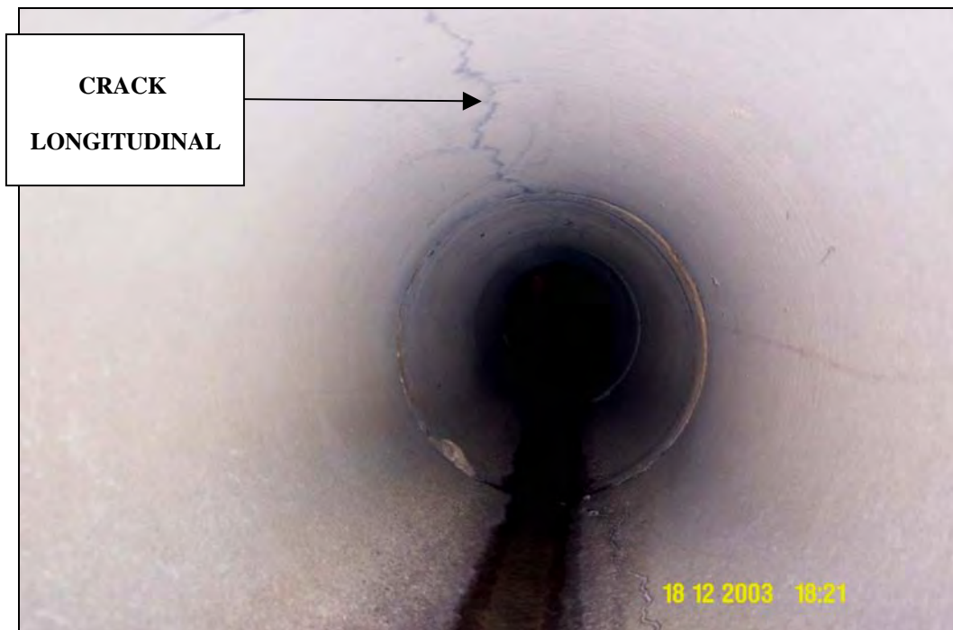
Crack runs along the axis of the pipe (parallel to the centerline)
