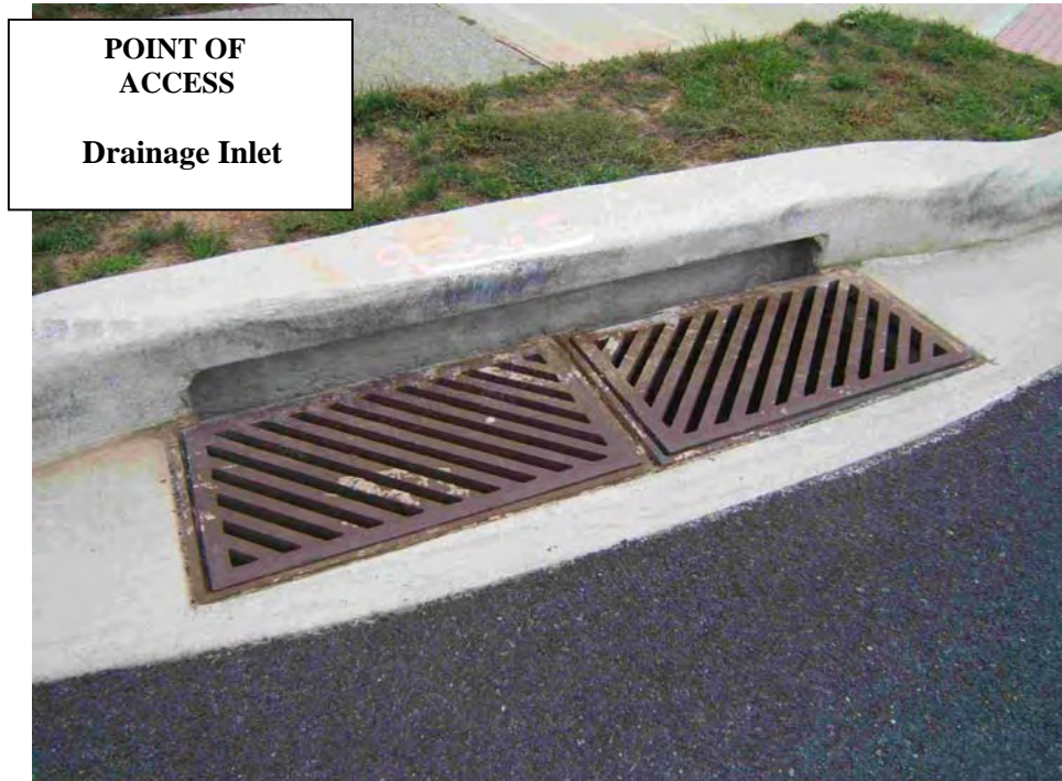
Double Grate Drainage Inlet.
