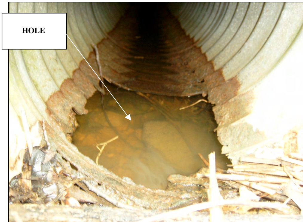
A visible hole in the pipe/structure wall from corrosion.
