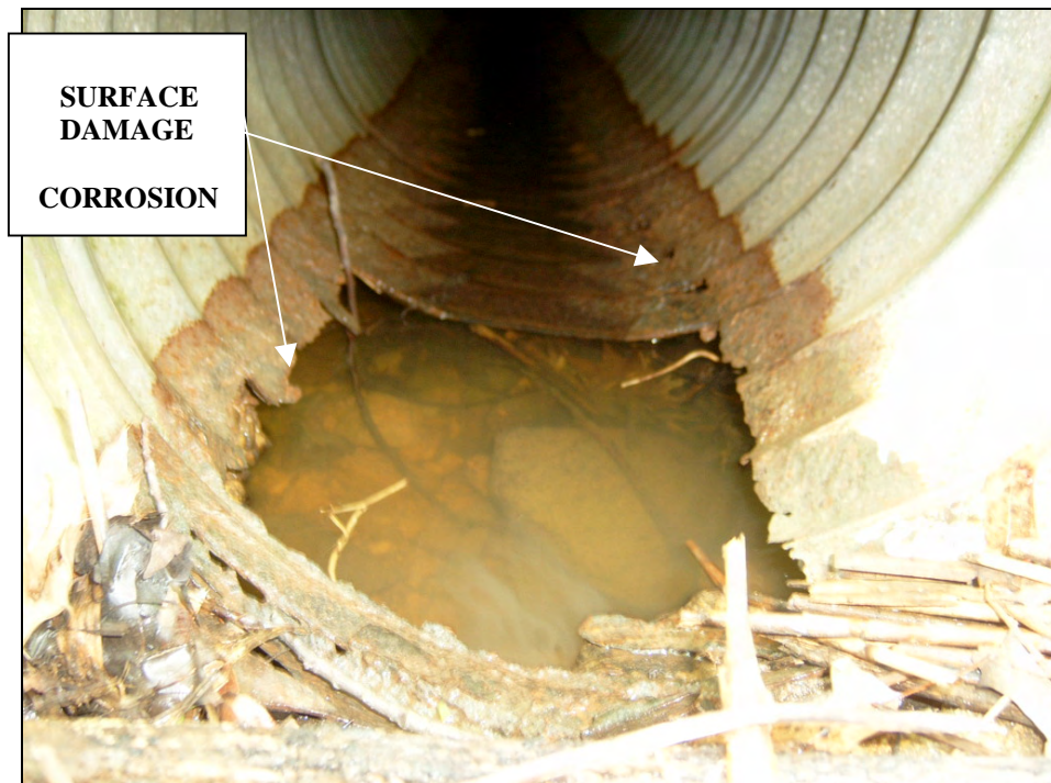
A visible loss of pipe material by corrosive attack.
