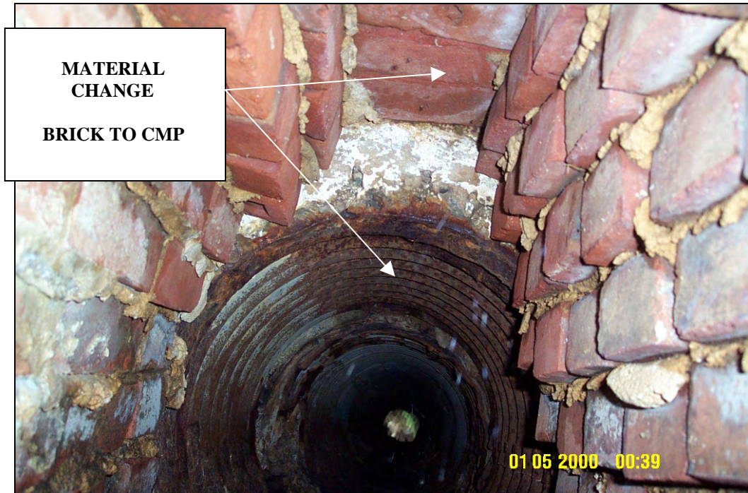
Material Change from Brick to CMP
