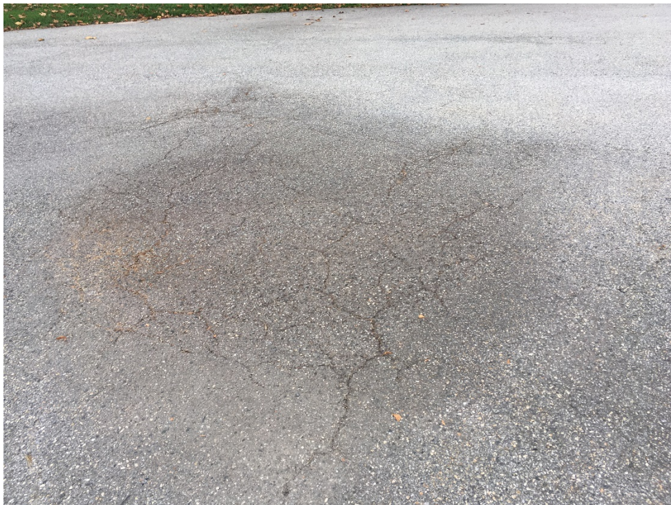
Photo 2 – Isolated cracking and surface depression in parking lot area
