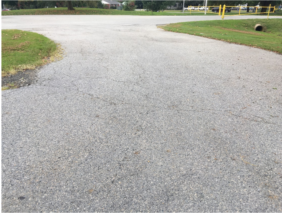
Photo 1 – Isolated alligator cracking in parking lot area
