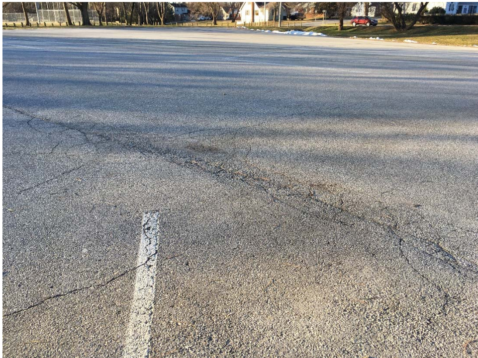
Photo 8 – isolated cracking near apparent pavement joint in middle of parking lot
