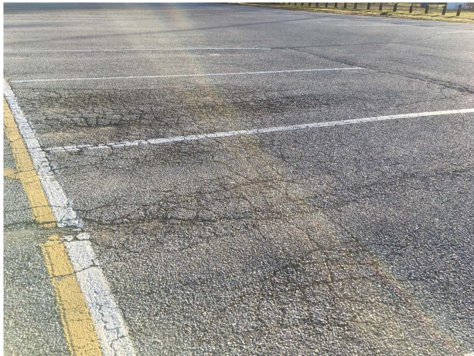
Photo 6 – moderate to severe alligator cracking
