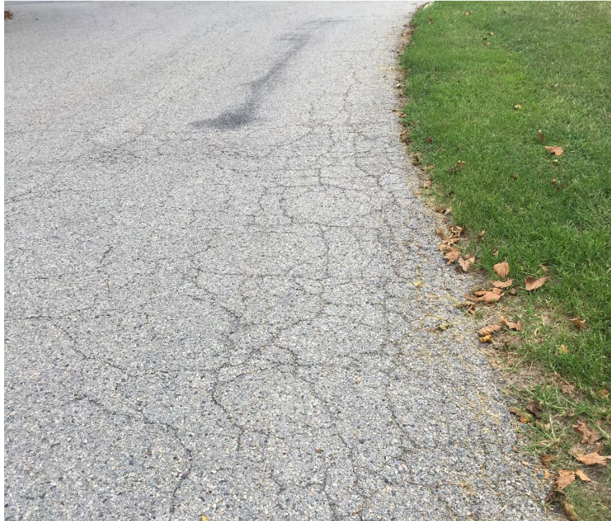
Photo 3 – Isolated alligator cracking in parking lot area
