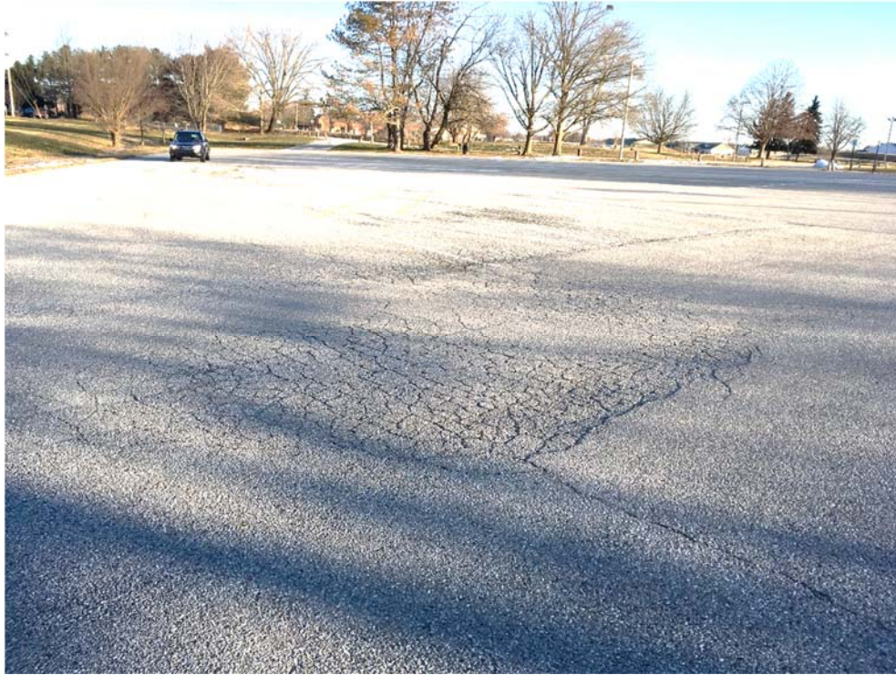
Photo 5 – moderate to severe alligator cracking
