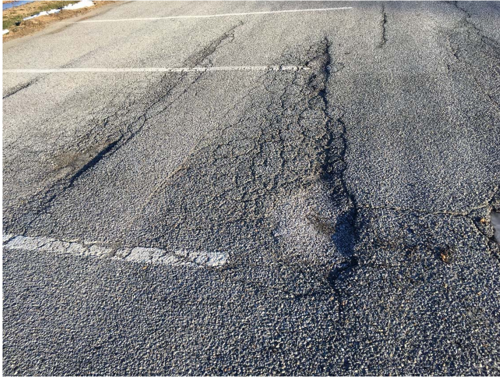
Photo 3 – potholes and moderate to severe cracking along west side of parking lot
