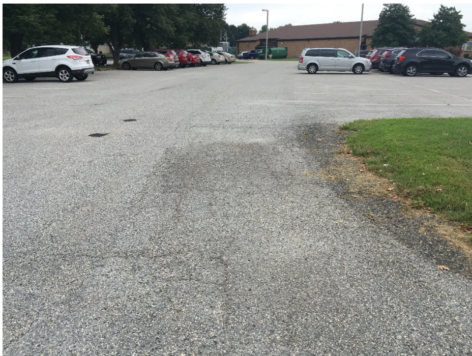
Photo 4 – Isolated alligator cracking in parking lot area
