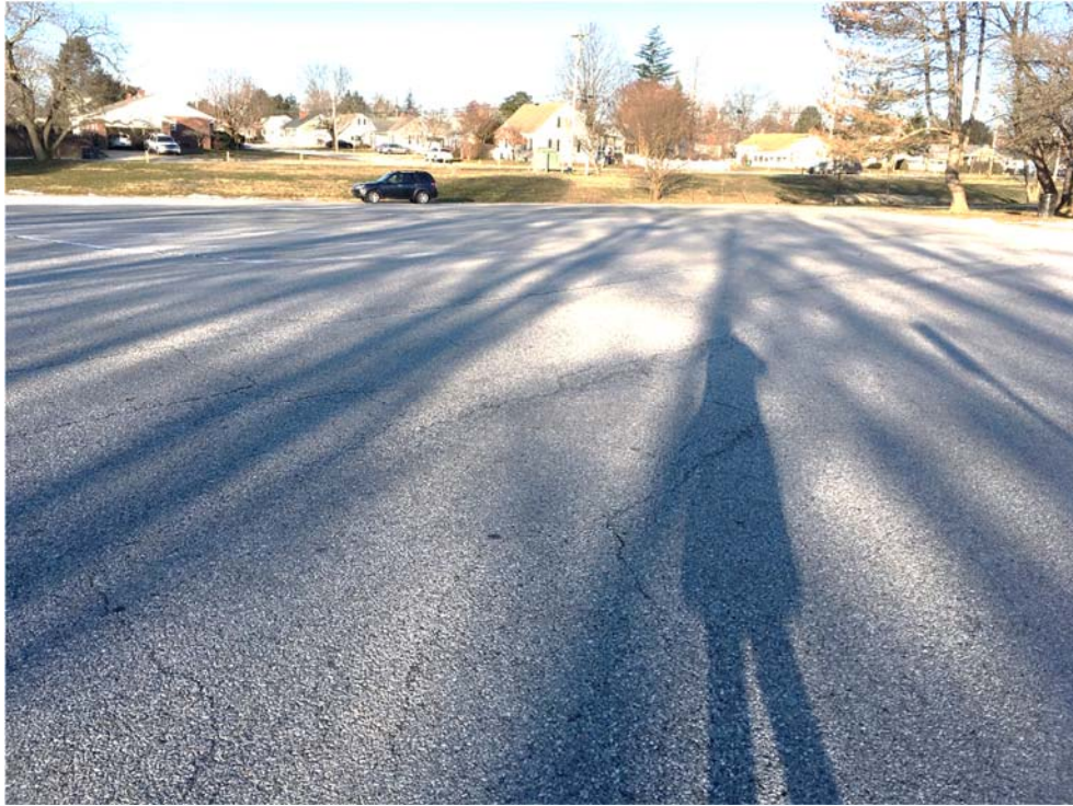
Photo 1 – Isolated cracks observed throughout majority of parking lot area
