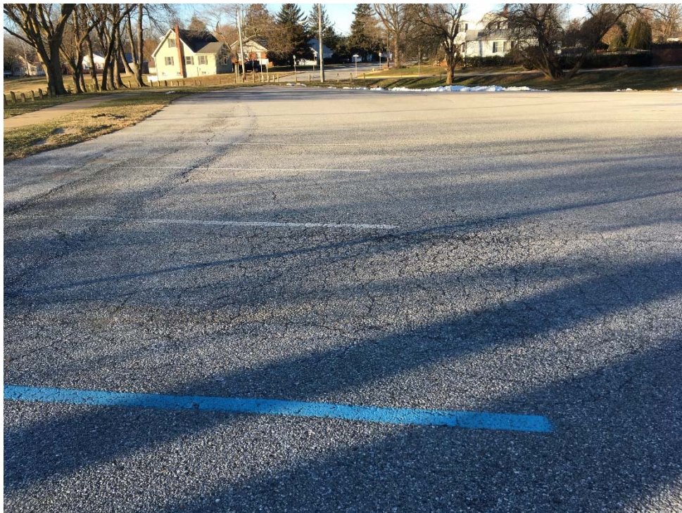
Photo 2 – moderate to severe alligator cracking and rutting along south end of west parking lot
