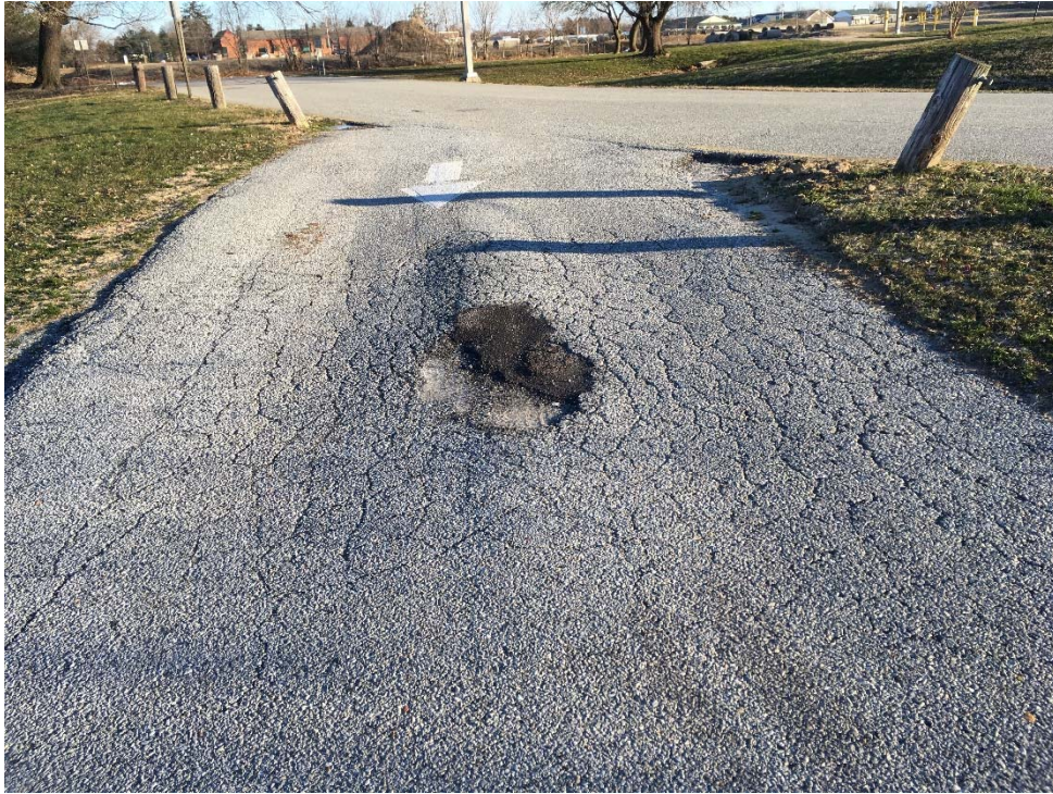
Photo 7 – pothole and moderate to severe alligator cracking at parking lot access drive
