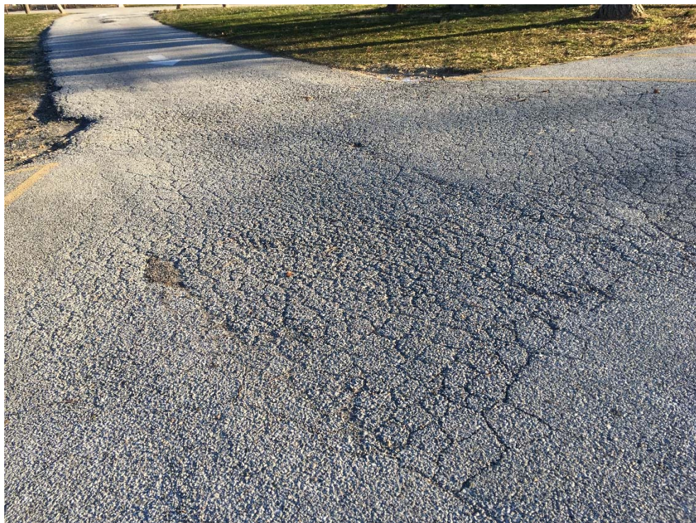
Photo 4 – severe alligator cracking near parking lot entrance
