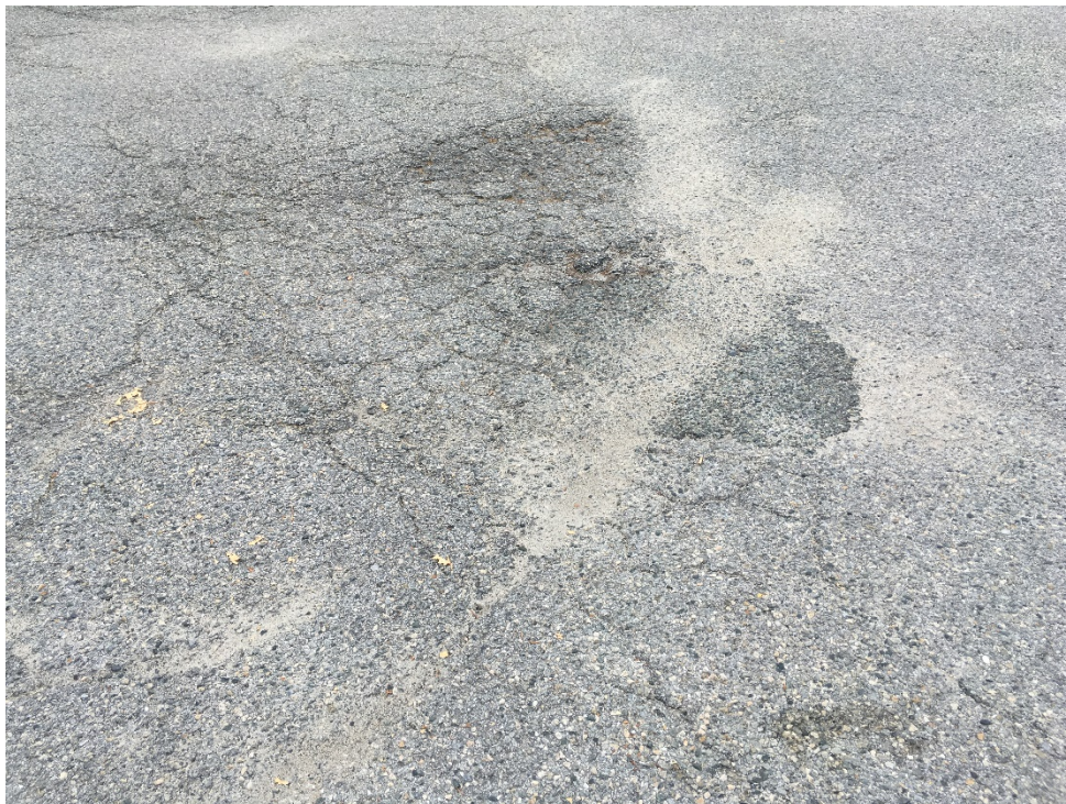
Photo 6 – Close up of cracking pavement deterioration from Photo 5 above
