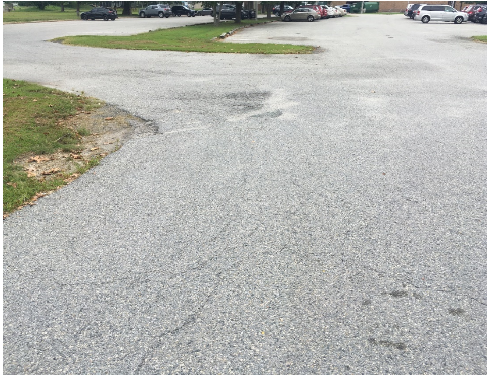
Photo 5 – Isolated alligator cracking and rutting in parking lot area
